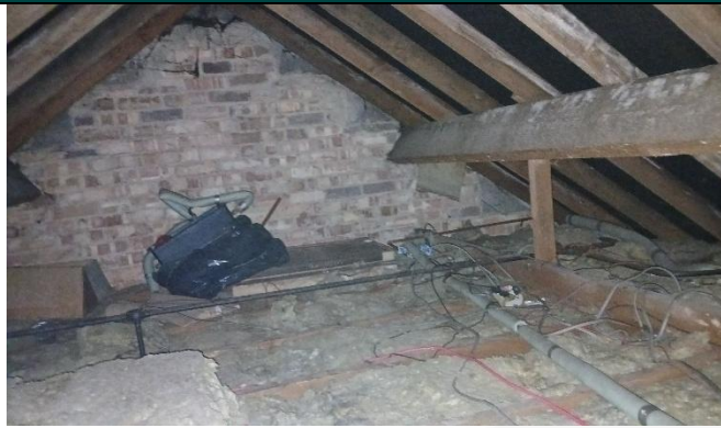
Figure 2 – L1 facing south
