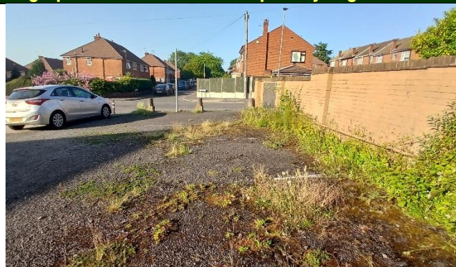
Figure 2 – southeastern corner of car park
