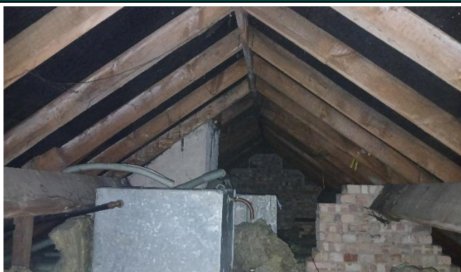
Figure 1 L1 facing north
