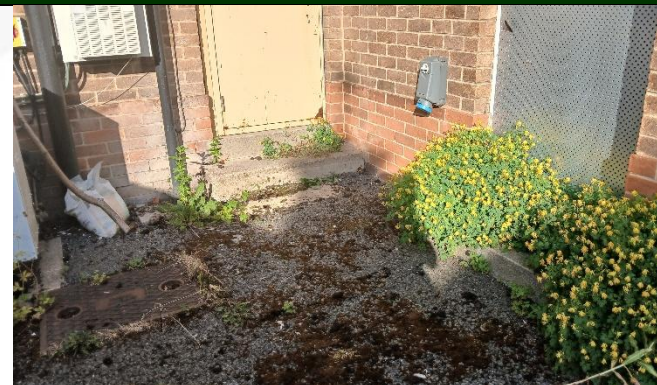
Figure 3 – western porch area
