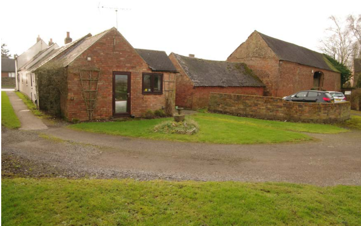
Figure 18: Northern side of the site Looking south. The threshing barn and stable are on the right. The office annex is in the foreground on the left. Main Street can be seen on the far left down the track
