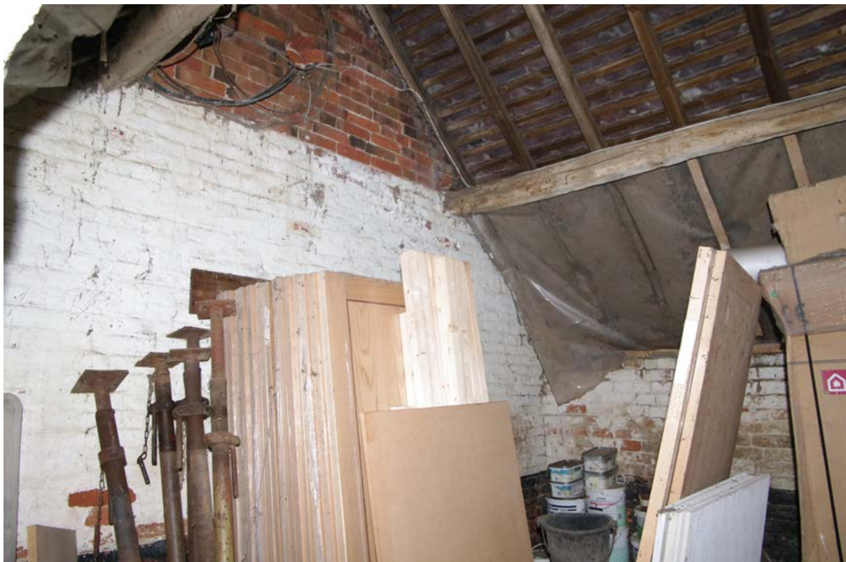
Figure 48: North-eastern stable, end wall with the threshing barn Looking north-west
