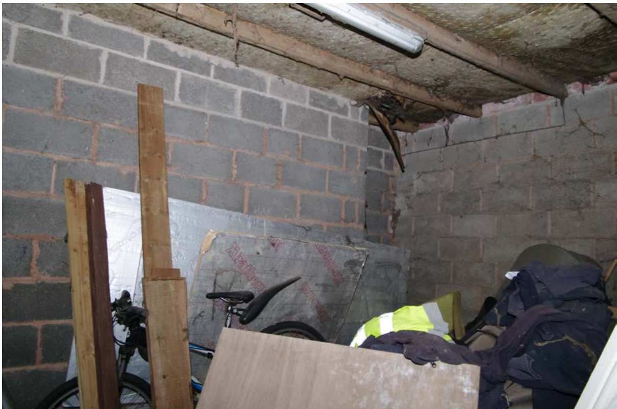
Figure 36: Threshing barn ground floor store to the east of the central doorway Looking east. The internal dividing walls are concrete blocks as are the lined external walls (to the right of this picture)
