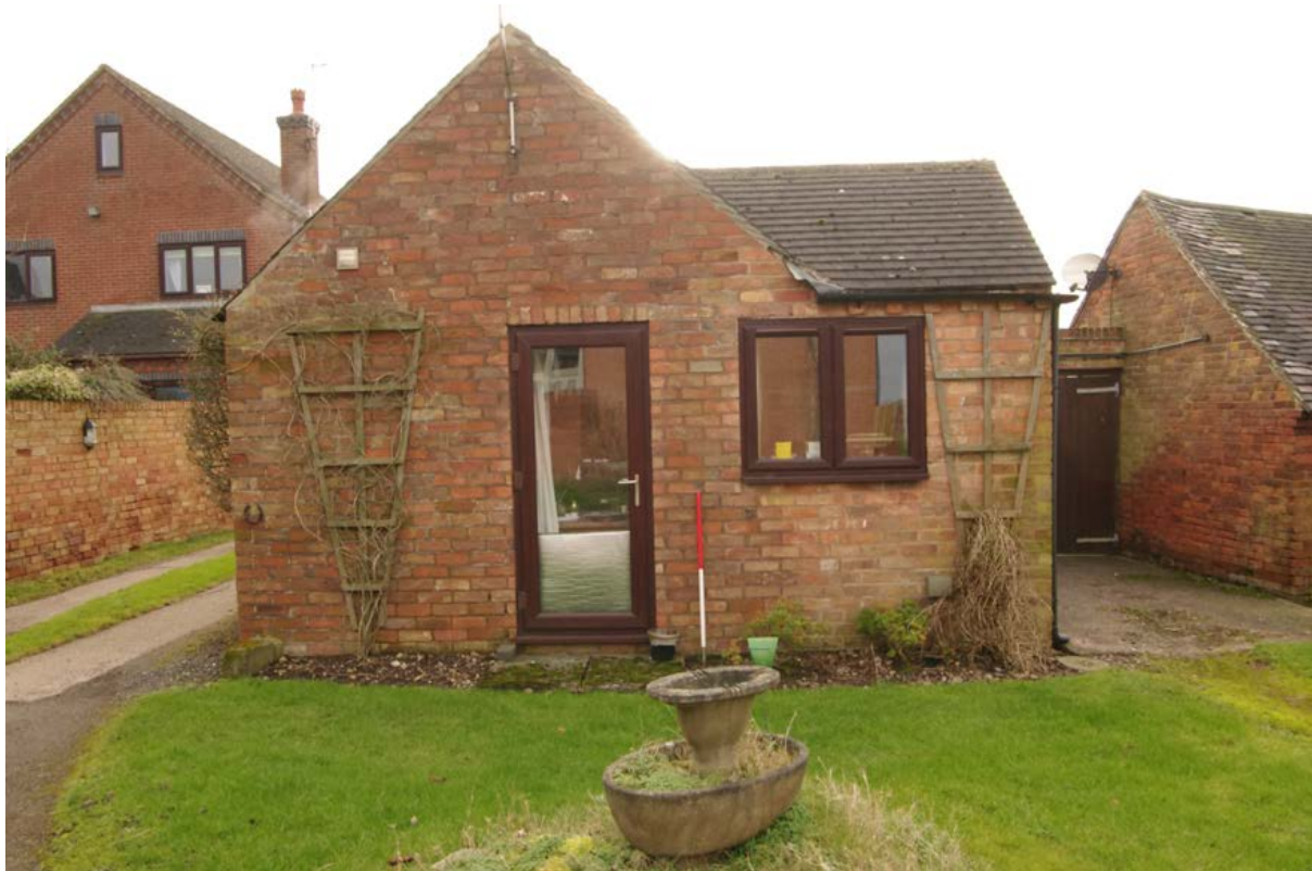
Figure 52: North-west facing elevation of the office annex Looking south-east. 1m scale. The north-eastern stable building is on the right
