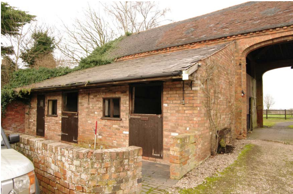
Figure 32: Stables built against the south-east facing elevation of the threshing barn
