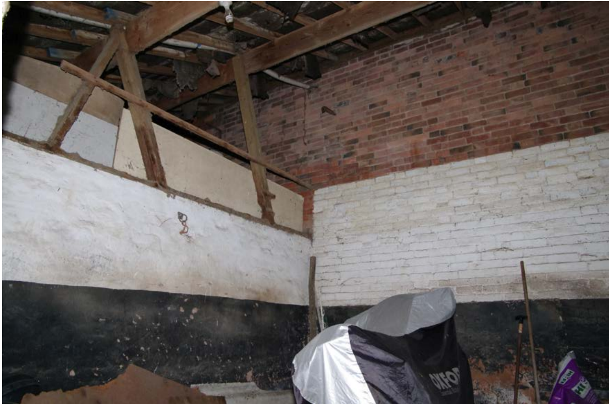
Figure 43: South-western stable roof structure Looking north-west. Threshing barn south-west facing wall on the right
