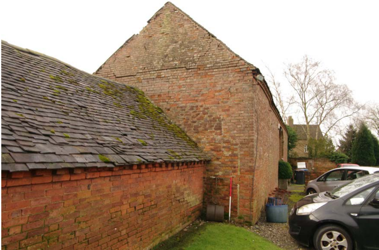
Figure 31: Threshing barn. North-east facing elevation
