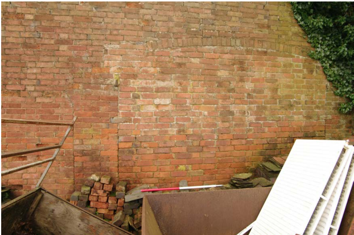
Figure 28: Threshing barn. Western end of the north-west facing elevation Note the wide opening above the 1m scale. There is evidence of another blocking to the left of this
