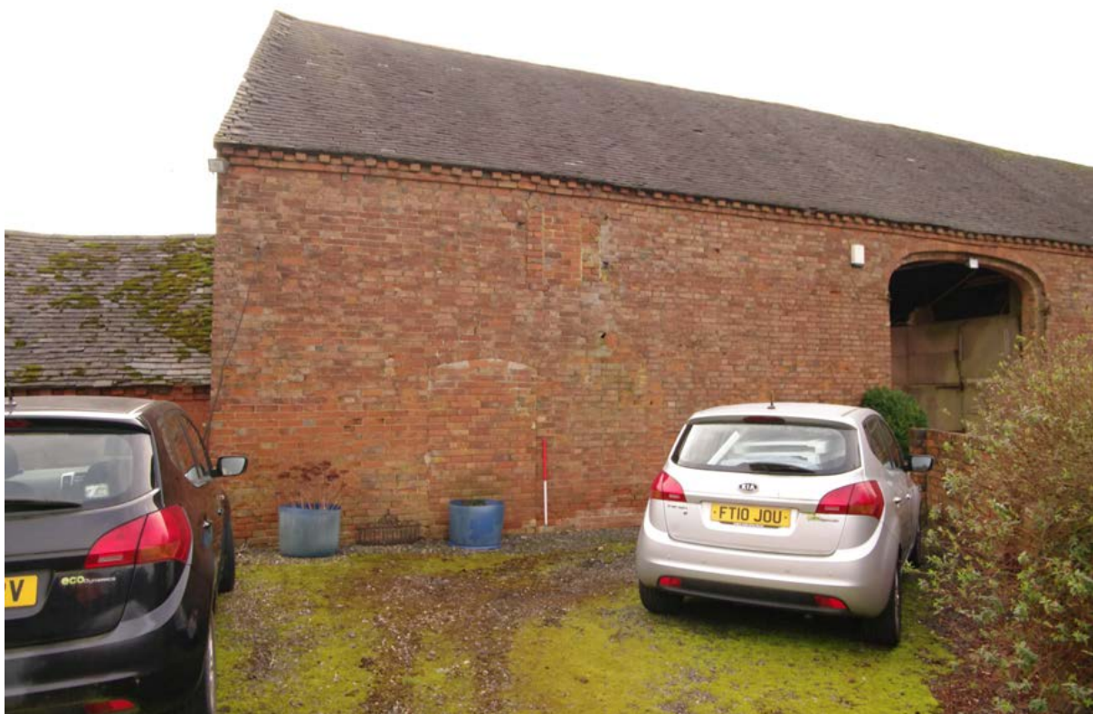
Figure 26: Threshing barn. Eastern end of the north-west facing elevation Note the blocked doorway to the left of the 1m scale. Another first floor window above the scale has been blocked
