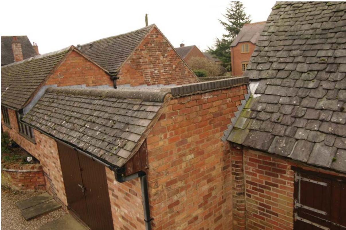
Figure 24: Flat-roofed section on the southern range
