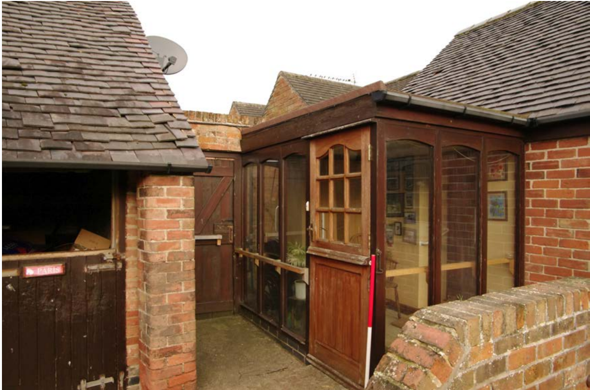
Figure 54: Porch attached to the south-west corner of the office annex Looking north-east. 1m scale. The small gables of the office can be seen above the porch. The corner of the north east stable is on the left
