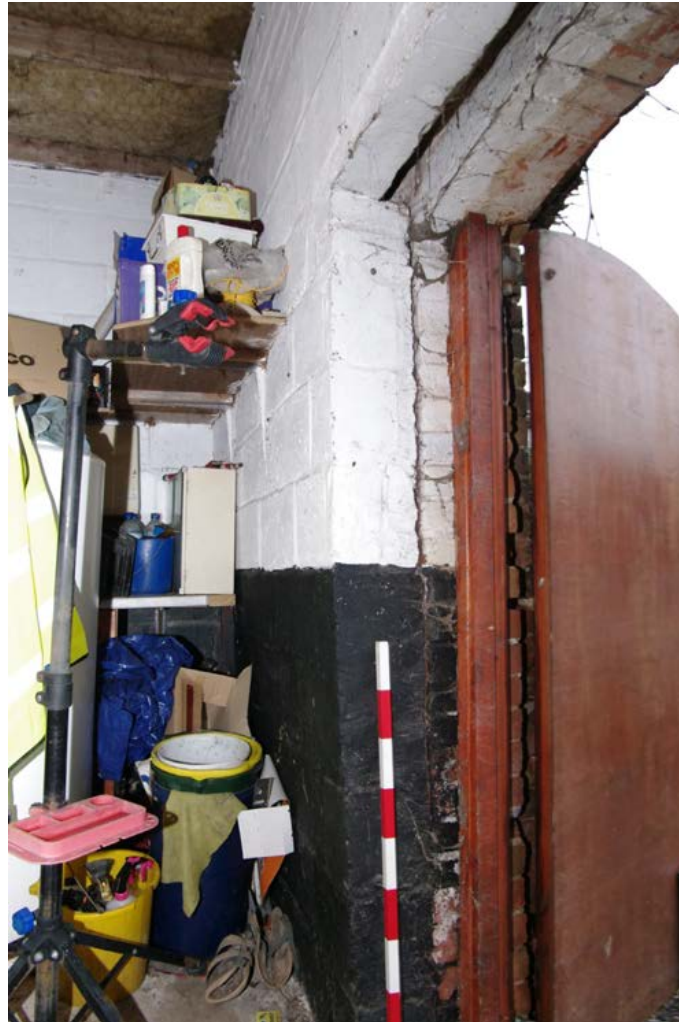
Figure 37: Threshing barn ground floor east end room
