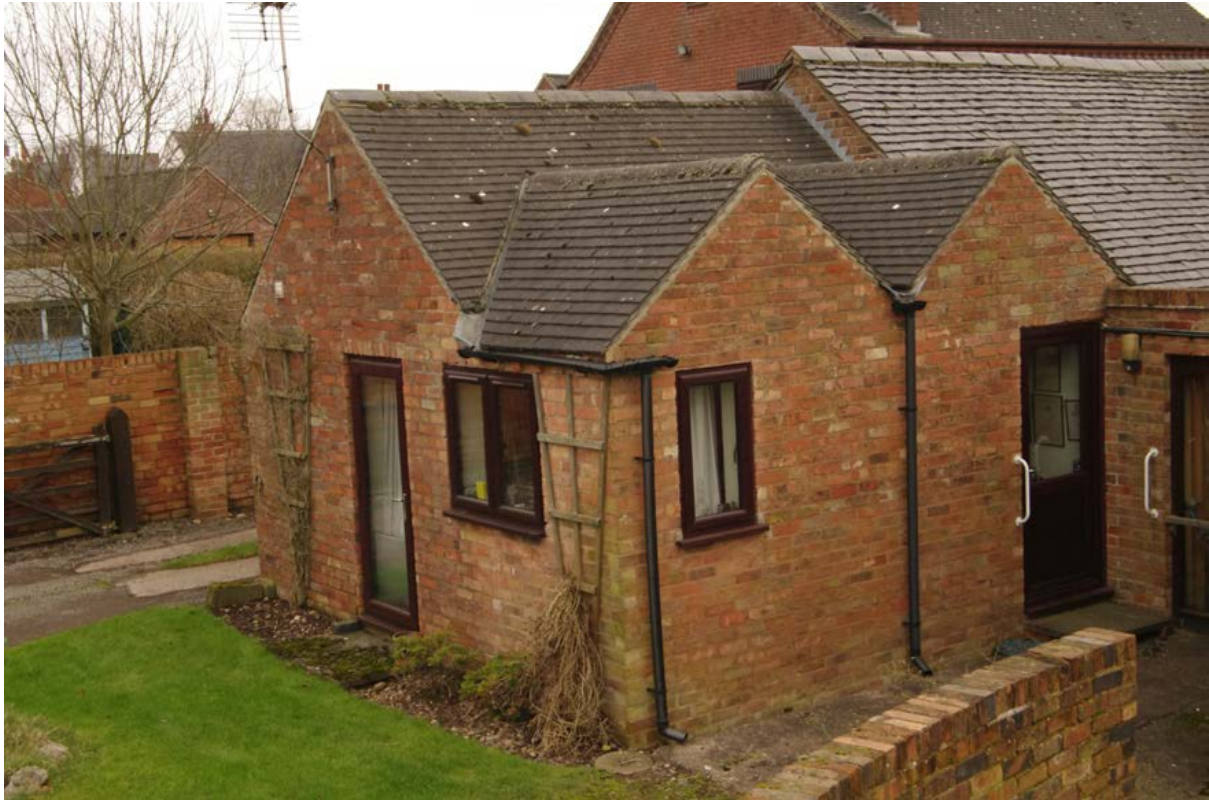
Figure 50: The office annex Looking south-east
