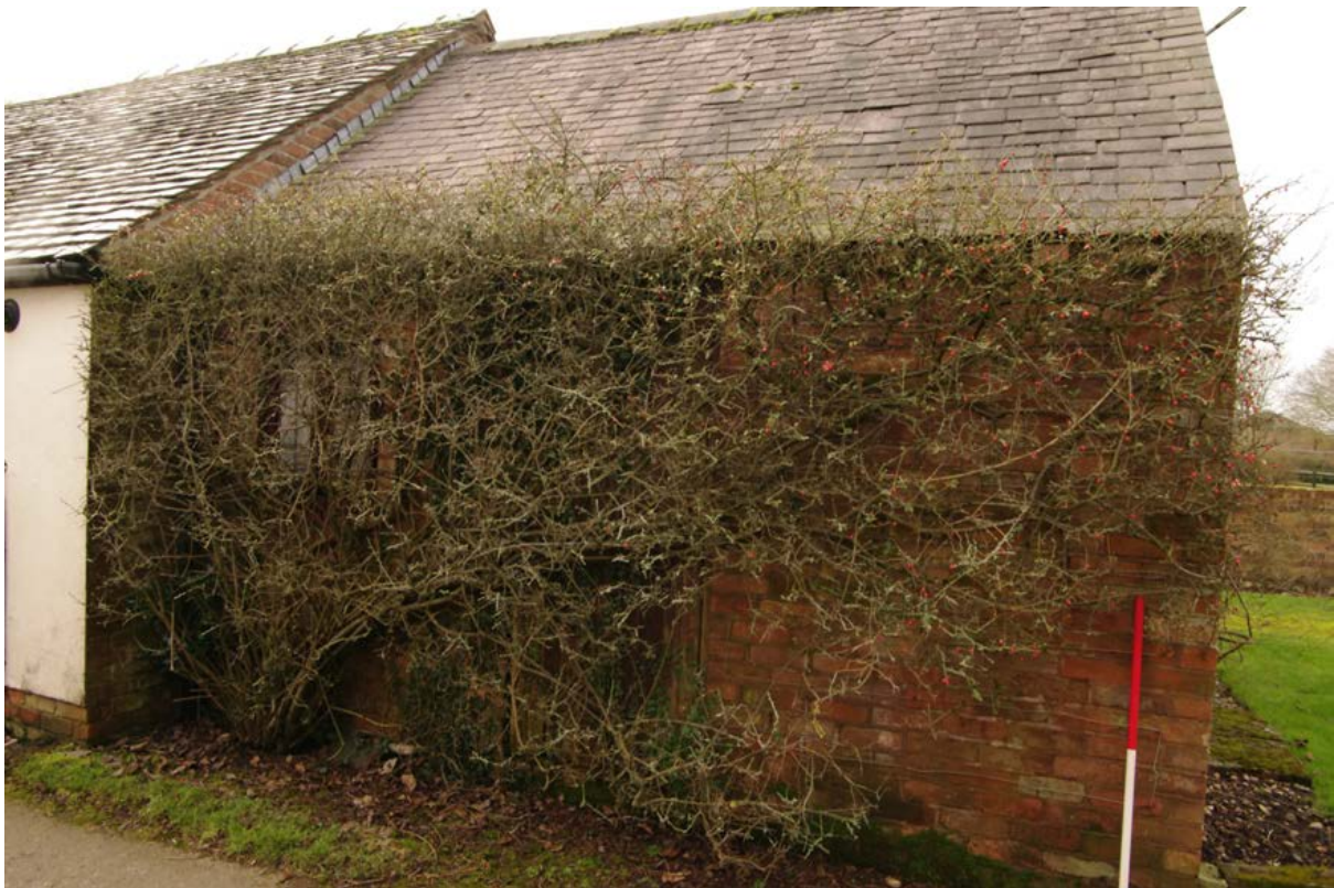
Figure 51: North-east facing elevation of the office annex Looking south-west. 1m scale. Note the obscured window and doorway behind the vegetation
