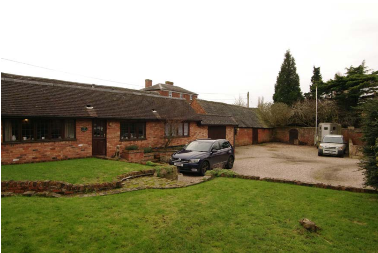
Figure 22: View of the yard looking south-west Note the low roofline above the black car which will be raised. Main Street runs behind these buildings
