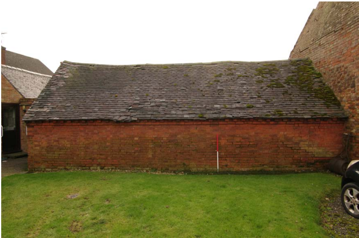
Figure 46: North-eastern stable, north-west facing elevation Looking south-east. 1m scale. Threshing barn on the right
