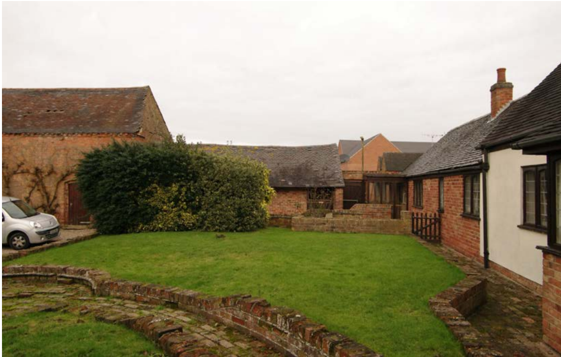
Figure 23: View of the yard looking NNE
