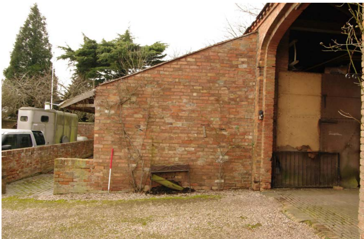
Figure 40: North-east facing elevation of south-western stable Looking south-west. 1m scale. Threshing barn on the right
