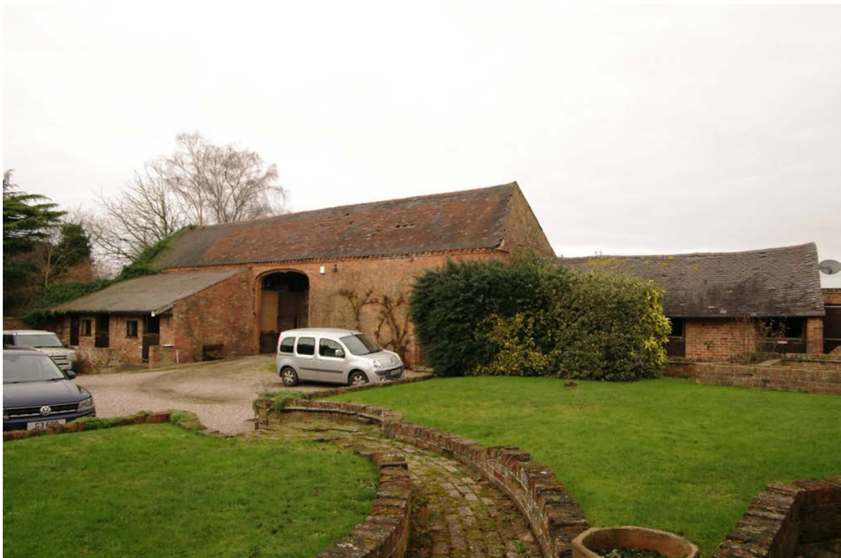
Figure 20: View of the yard looking north-west Looking towards the threshing barn and the two attached stables
