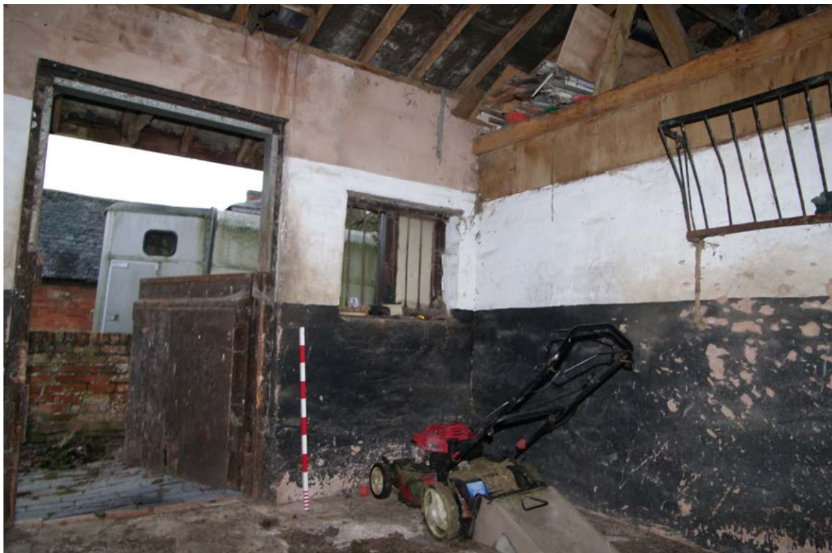
Figure 42: South-western stable building Looking south. 1m scale
