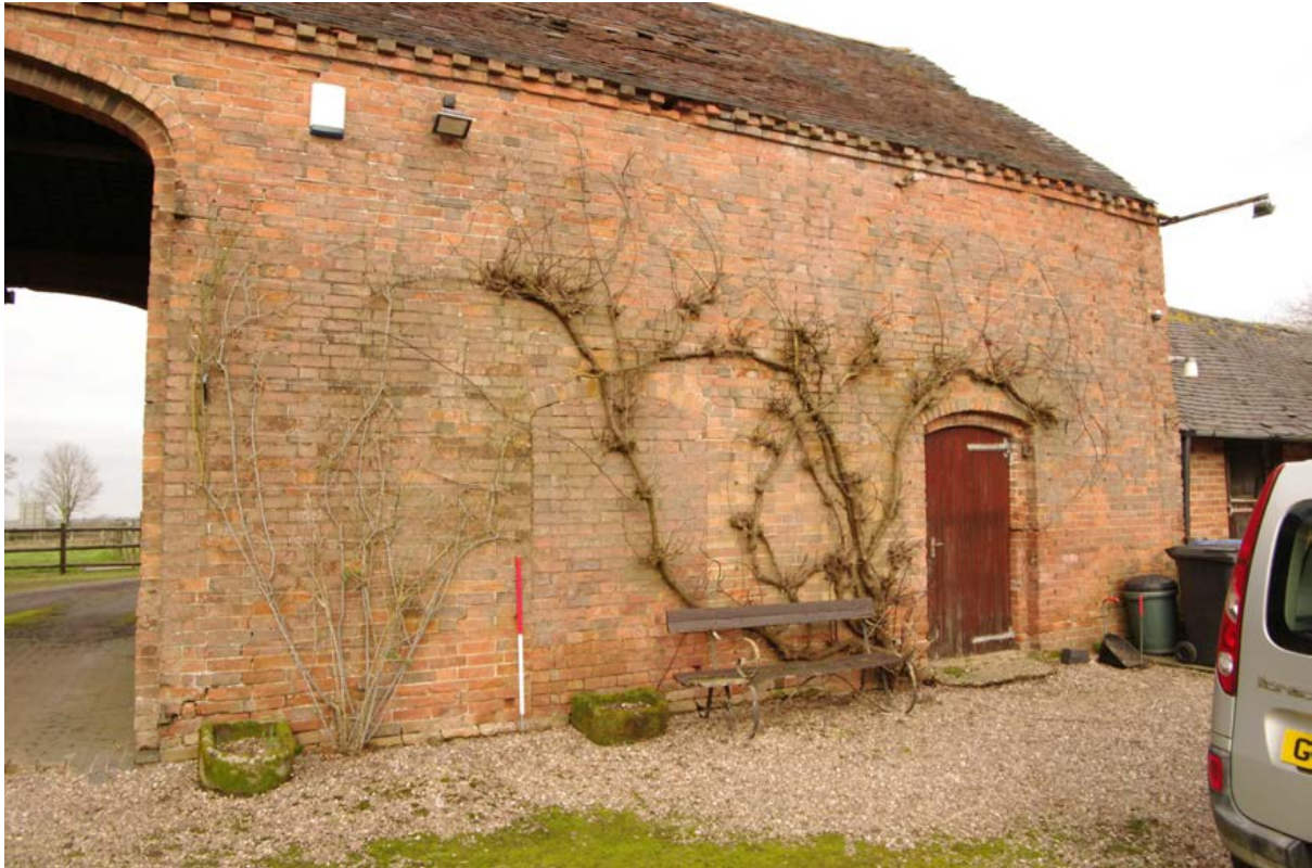
Figure 33: Threshing barn. Eastern end of the south-east facing elevation Looking north. 1m scale to the right of a blocked doorway
