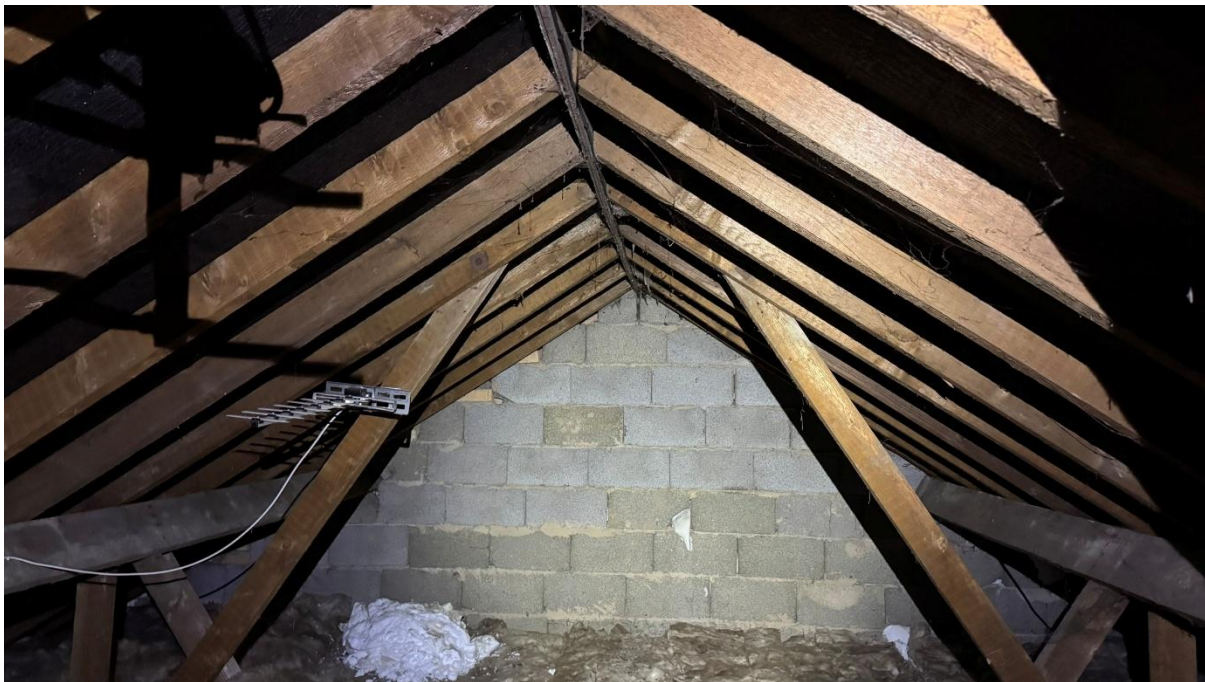
Photograph 6: The internal void of the dwelling, showing the open and uncluttered space.
