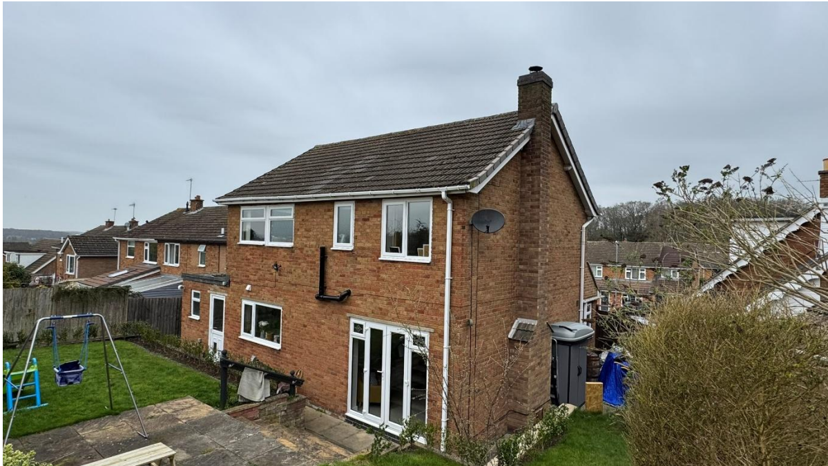
Photograph 3: The dwelling taken from the south-east, showing the chimney on the eastern gable.
