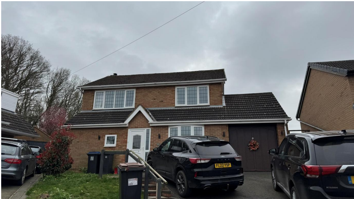
Photograph 1: The dwelling, taken from the north, showing the two-storey height with single storey front extension and garage on the west, with interlocking tile roof covering.
