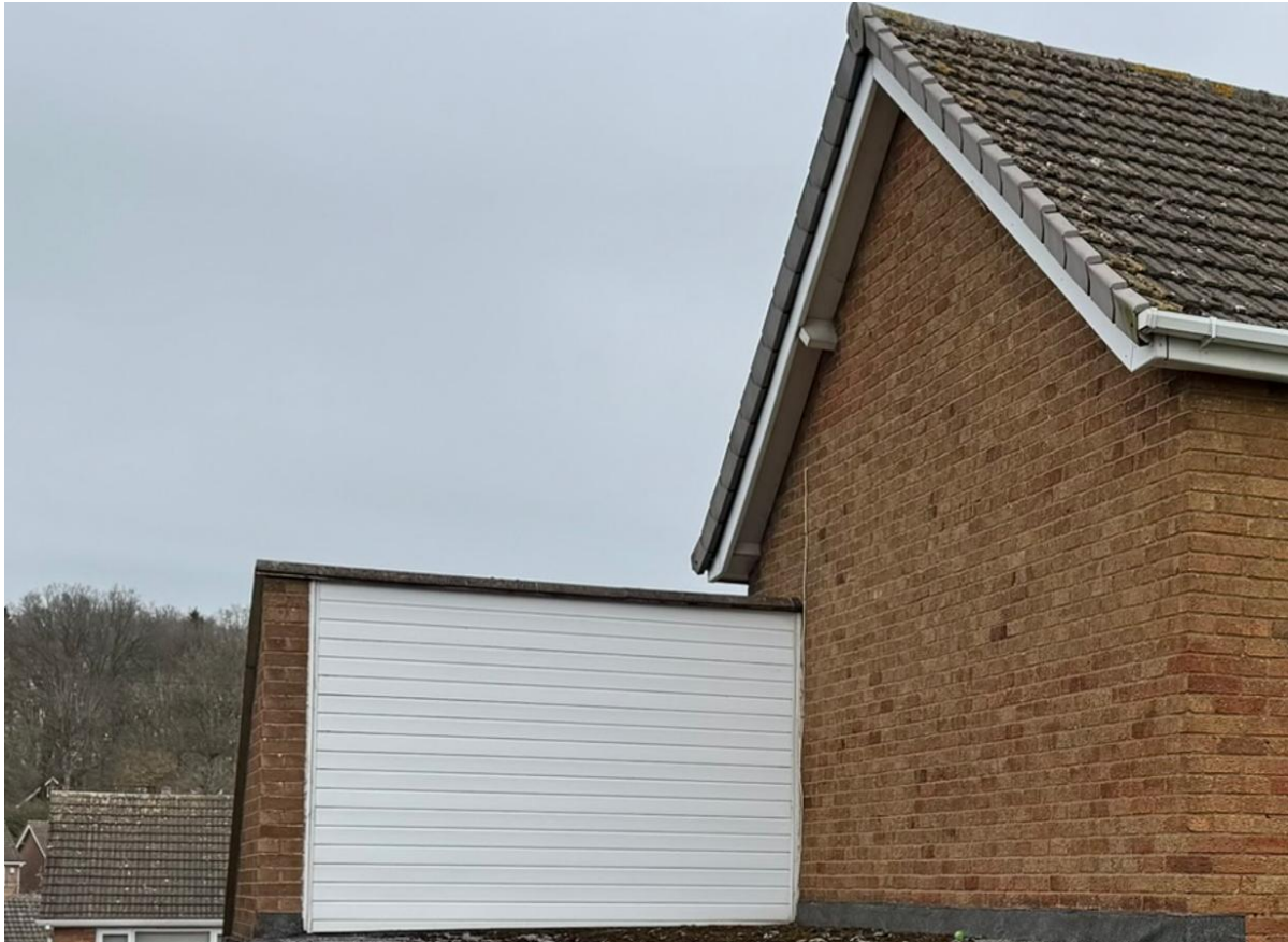
Photograph 11: The well fitted uPVC weatherboard and soffit box on the western end, where development works are planned.
