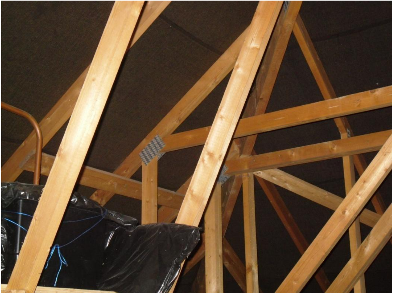
Loftspace image: preformed wooden truss construction
