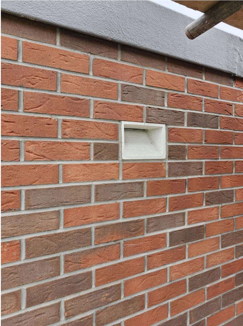
FIGURE 8 - X1 BAT BOX INSTALLED ON NORTH ELEVATION
