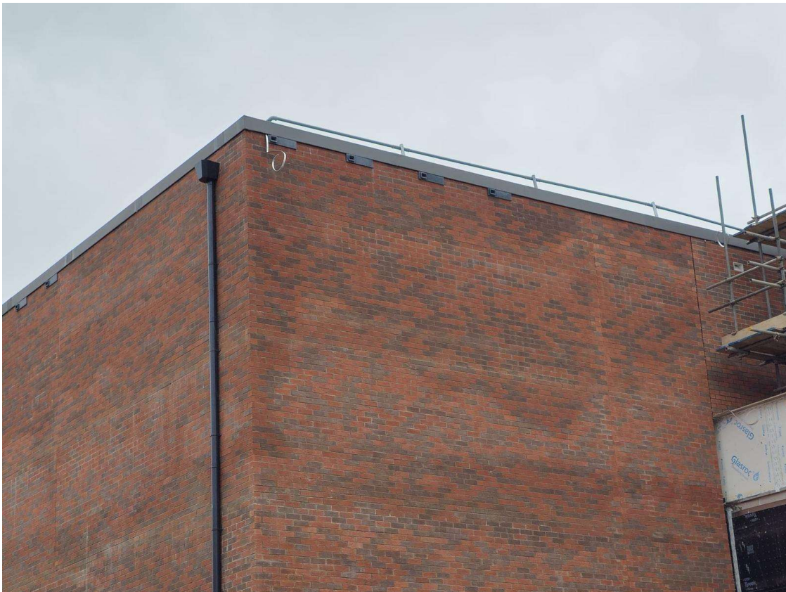
FIGURE 1 - X4 SWIFT BOXES INSTALLED ON NORTH ELEVATION
