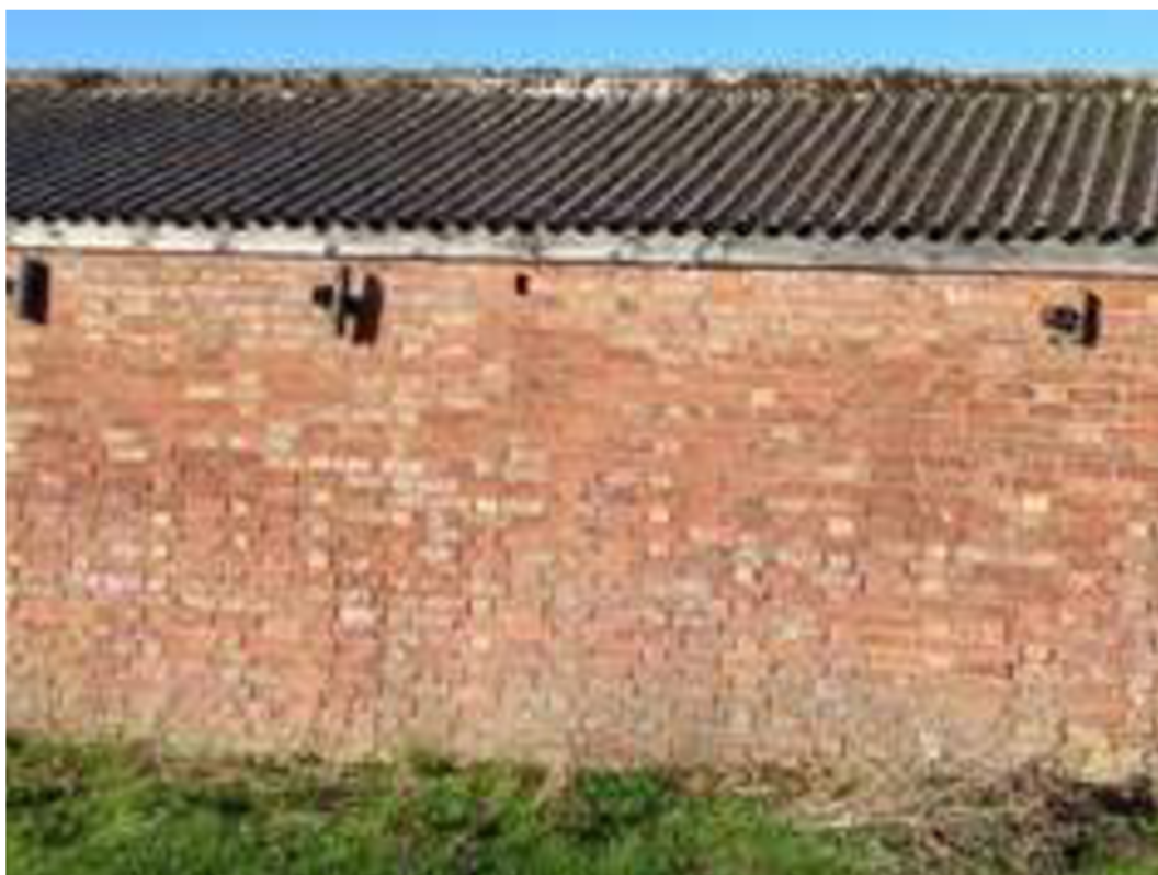
Photo 6—The majority of the barn roof.
