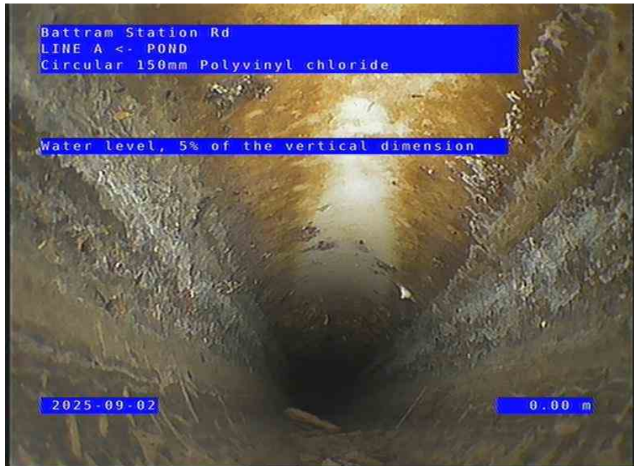
LINE A X_cf1efcf2-1ca3-4c33-a48e-0ccc09262177_20250902_102018_725.jpg, 00:00:01, 0.00 m
