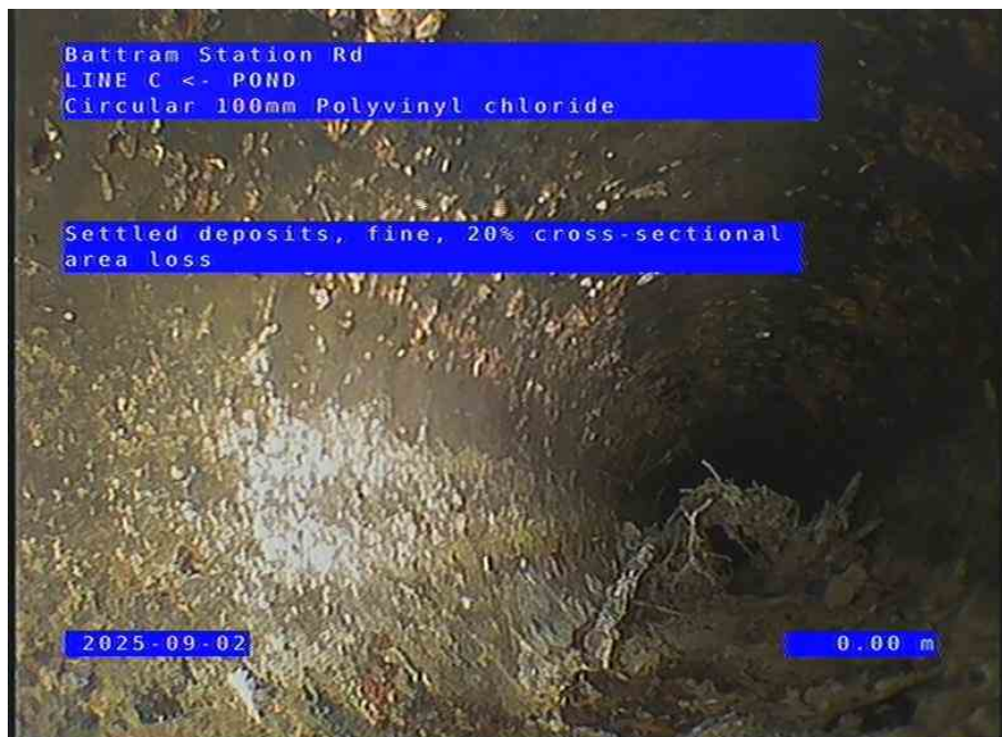
LINE C X_c3014773-c768-461f-9878-2f5bbd0940dc_20250902_104328_078.jpg, 00:00:05, 0.00 m
