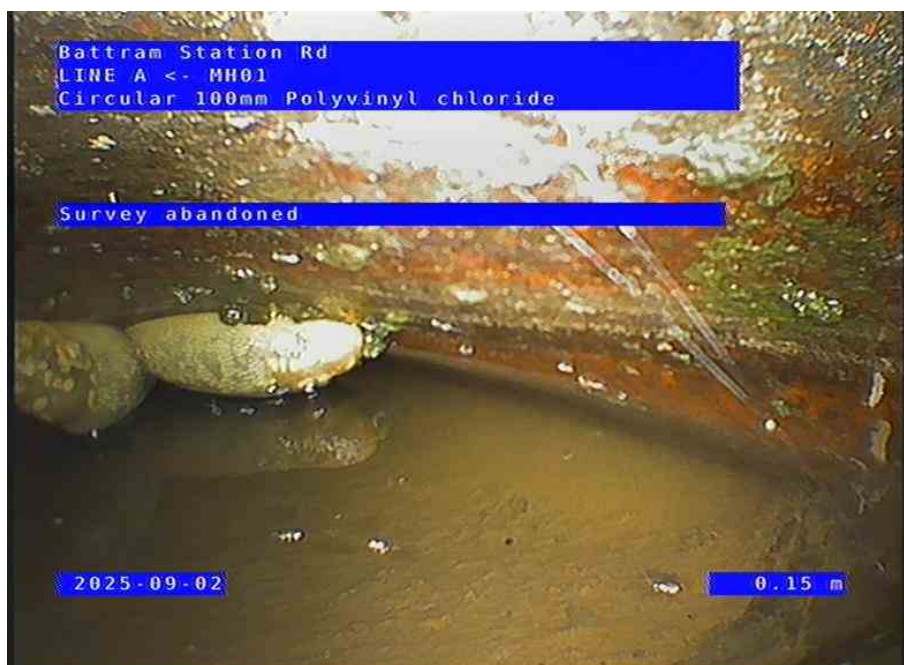
LINE A X_d7293cbc-3eed-472e-938c-4a3ae21417c3_20250902_141418_442.jpg, 00:00:25, 0.15 m
