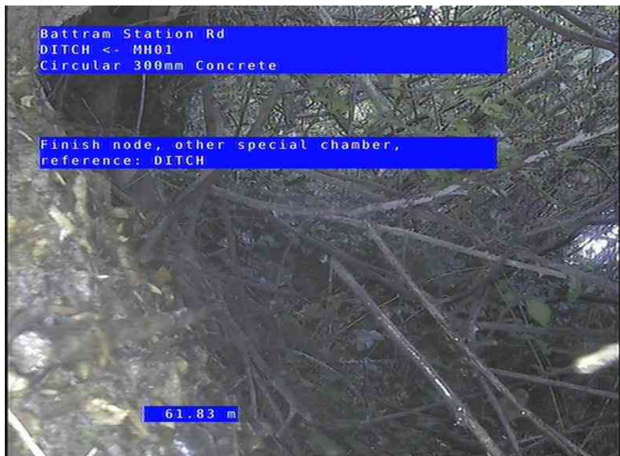
DITCHX_933d433e-9aeb-4cd7-8f7a-07ca98fae226_20250903_081647_419.jpg, 00:06:04, 61.83 m Finish node, other special chamber, reference: DITCH
