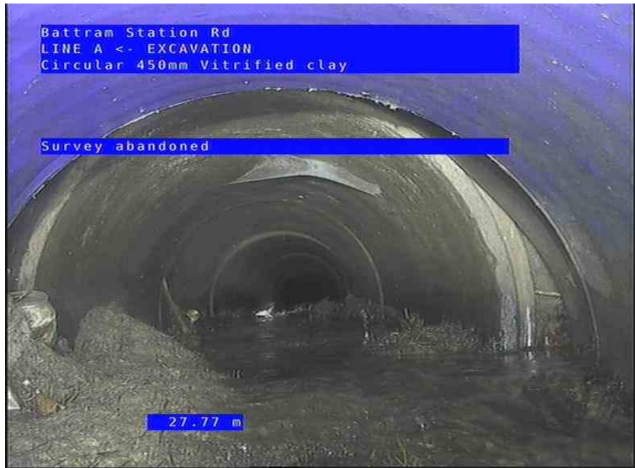
LINE A X_d2c3d344-737e-4a30-a9cb-1e3beb534973_20250903_105954_916.jpg, 00:02:17, 27.77 m Survey abandoned
