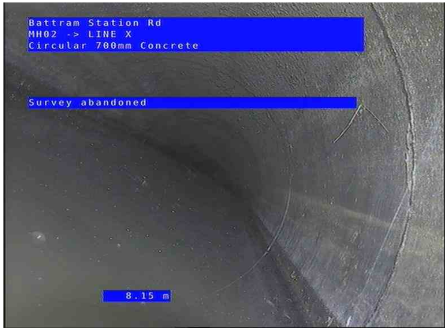
MH02X_75d770fe-fdf9-40a5-a393-c7de2ec813ae_20250903_091112_745.jpg, 00:01:32, 8.15 m Survey abandoned
