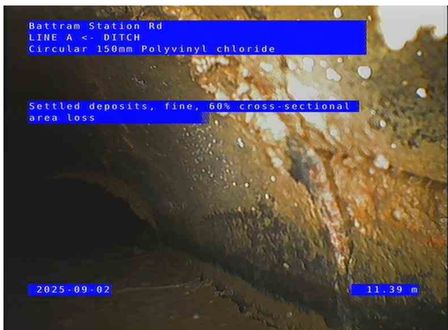
LINE A X_8388b26b-17da-4f5f-b9f3-3e3f27577893_20250902_111542_172.jpg, 00:01:28, 11.39 m
