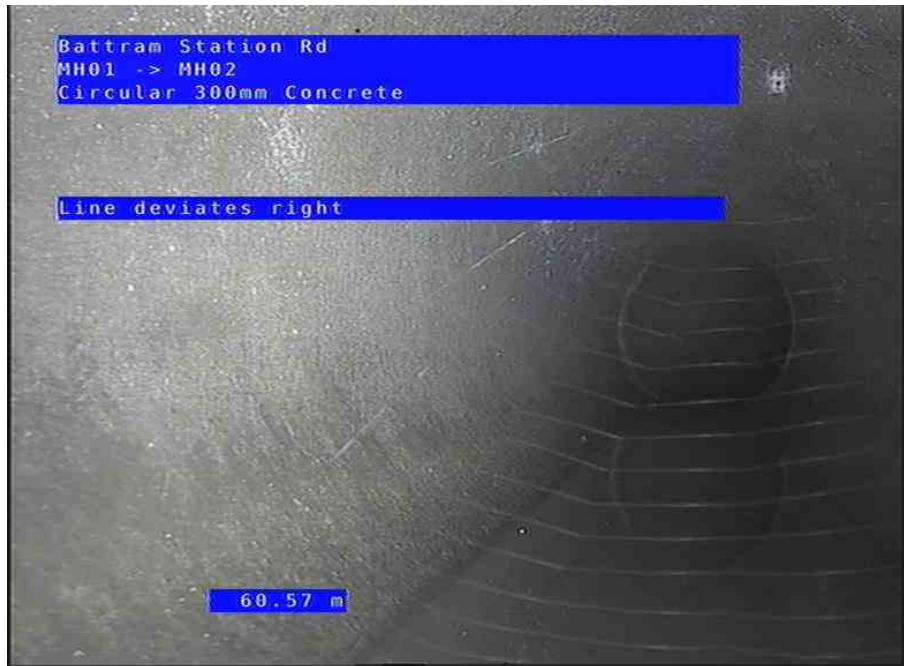
MH01X_9fd05cab-25d8-4c53-b640-1a868aa35fb0_20250902_143529_912.jpg, 00:04:31, 60.57 m Line deviates right
