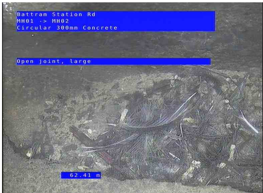
MH01X_f7970d14-b9bb-4be4-92c5-e2925fda31d5_20250902_143601_040.jpg, 00:04:57, 62.41 m Open joint, large
