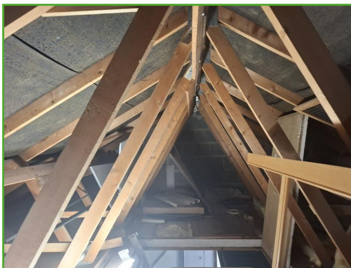
Picture 2: Internal view of the detached garage
