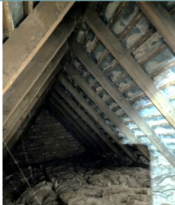
Plate 5: View of 1c roof void gable end via the small hole adjacent to the chimney breast only.
