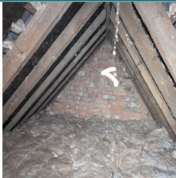
Plate 3: View of 1b roof void.
