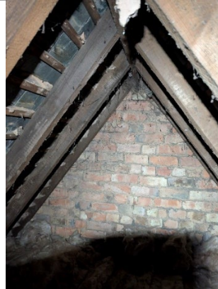
Plate 2: View of the 1a roof void gable end.
