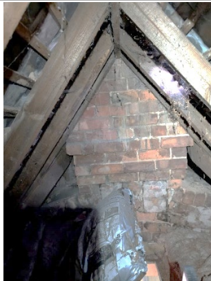
Plate 1: View of the chimney breast showing access to 1b and 1c loft spaces and loft hatch access point in the 1a roof void.
