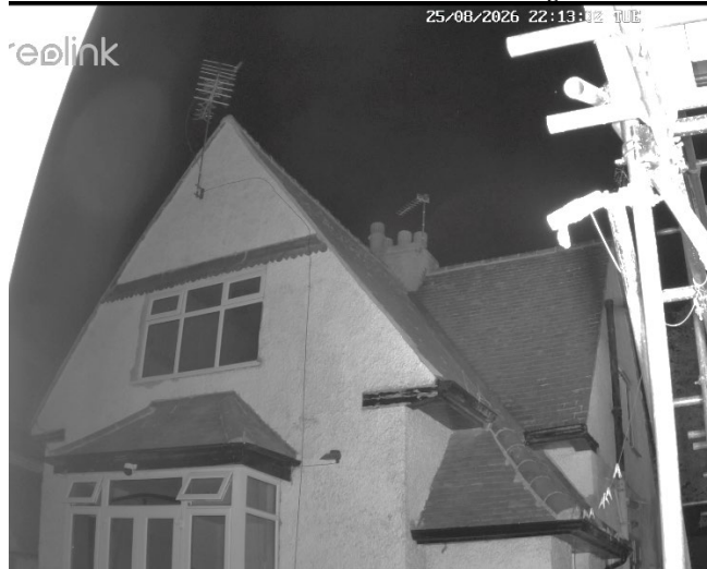
Plate 3. View of the rear of the main house looking northwest - NVA vantage point.
