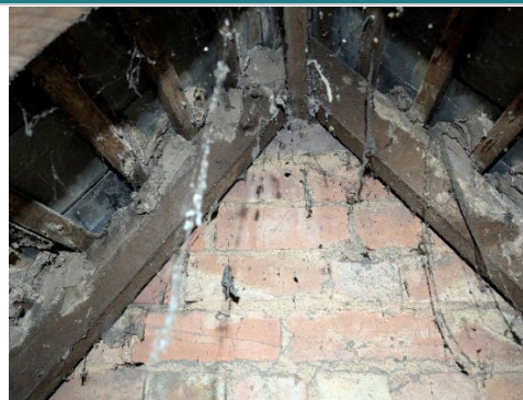
Plate 4: View of the 1b roof void gable end.
