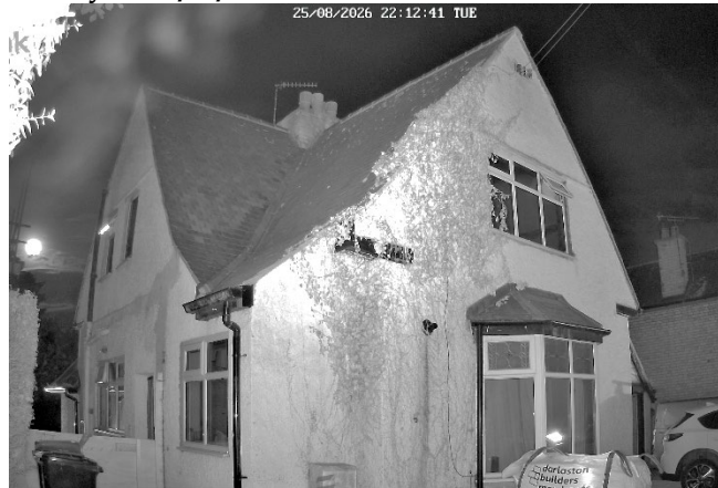
Plate 1. View from Front of main house looking southwest - NVA vantage point.
