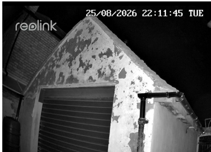
Plate 5. View of the rear garage and open soffit - NVA vantage point.
