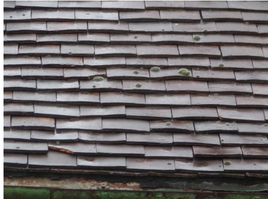
Picture 6: typical of roof on listed building
