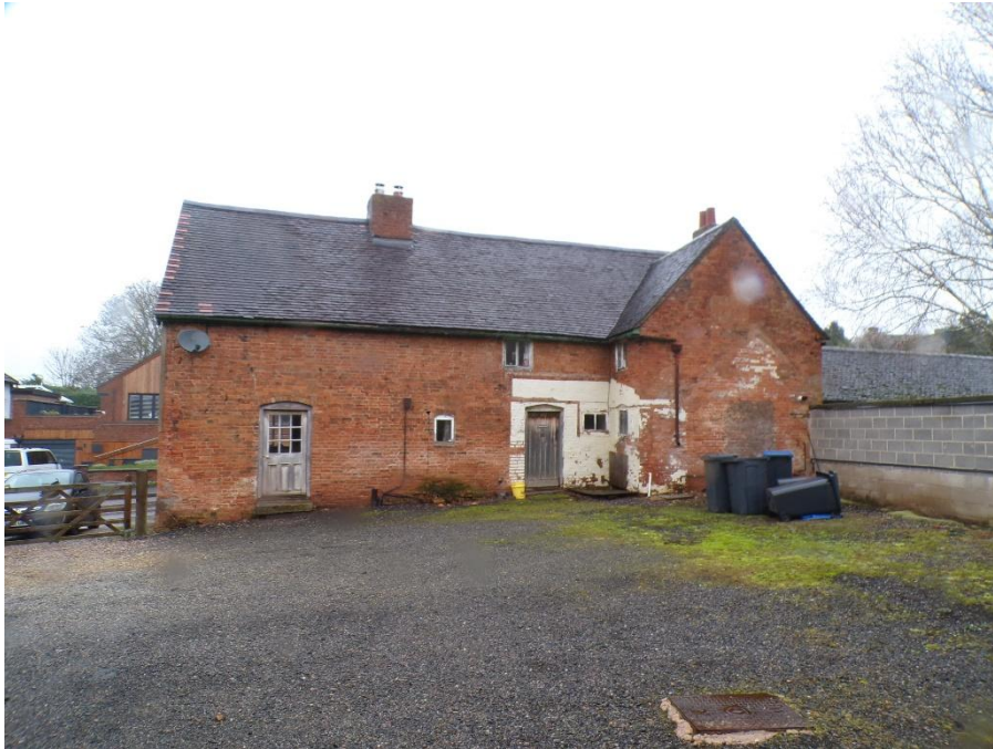
Picture 5: Rear of listed building with bat roost potential
