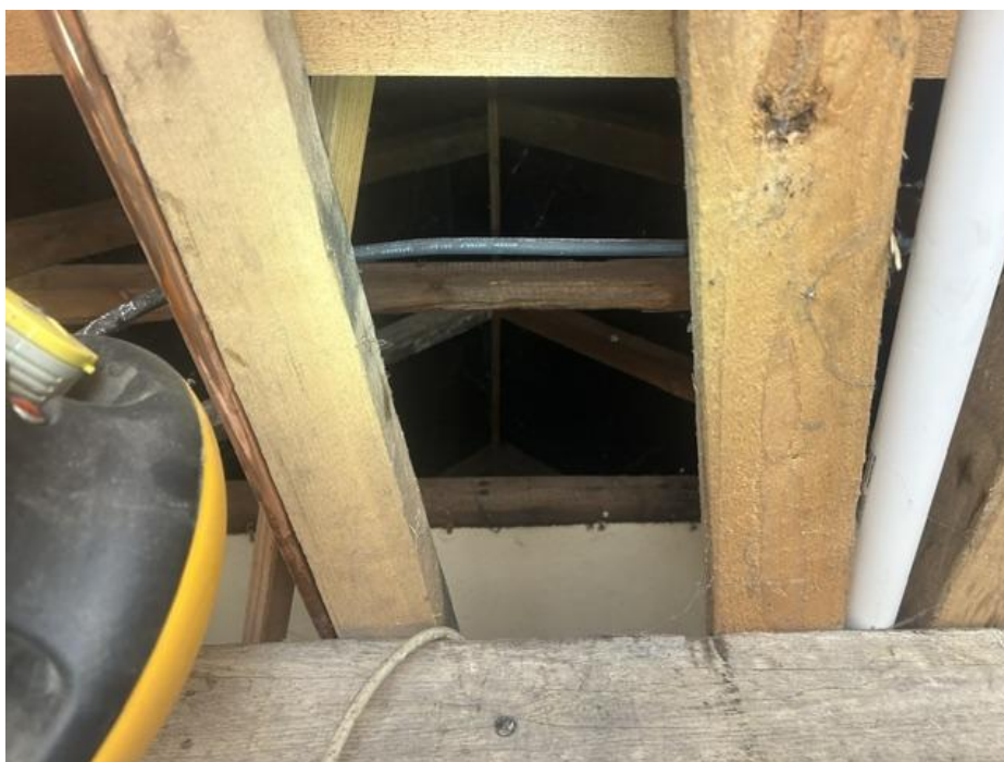
Figure 15 – Internal loft space B2
