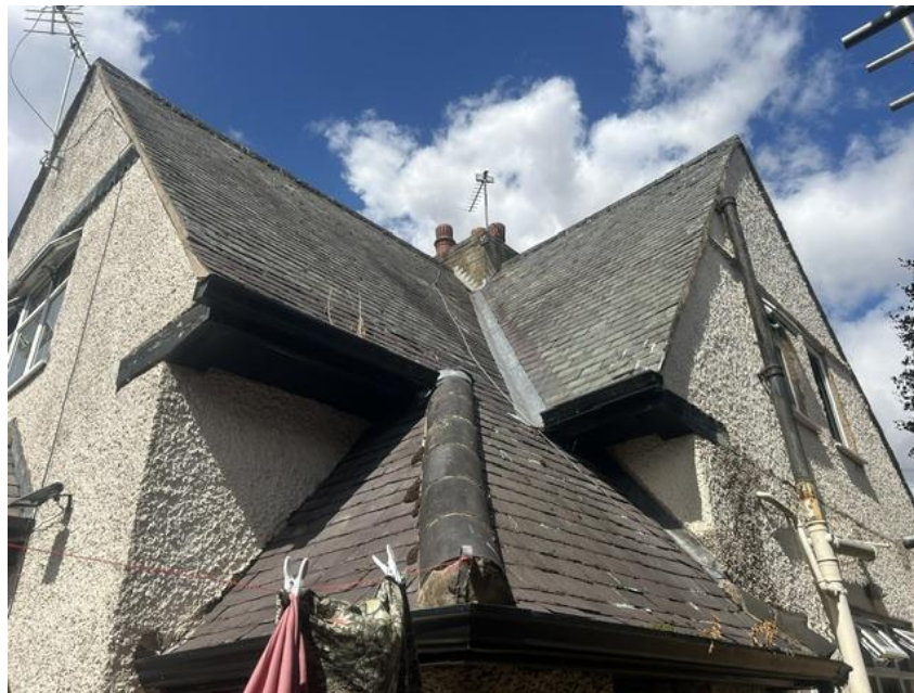
Figure 7 – Damaged mortar
