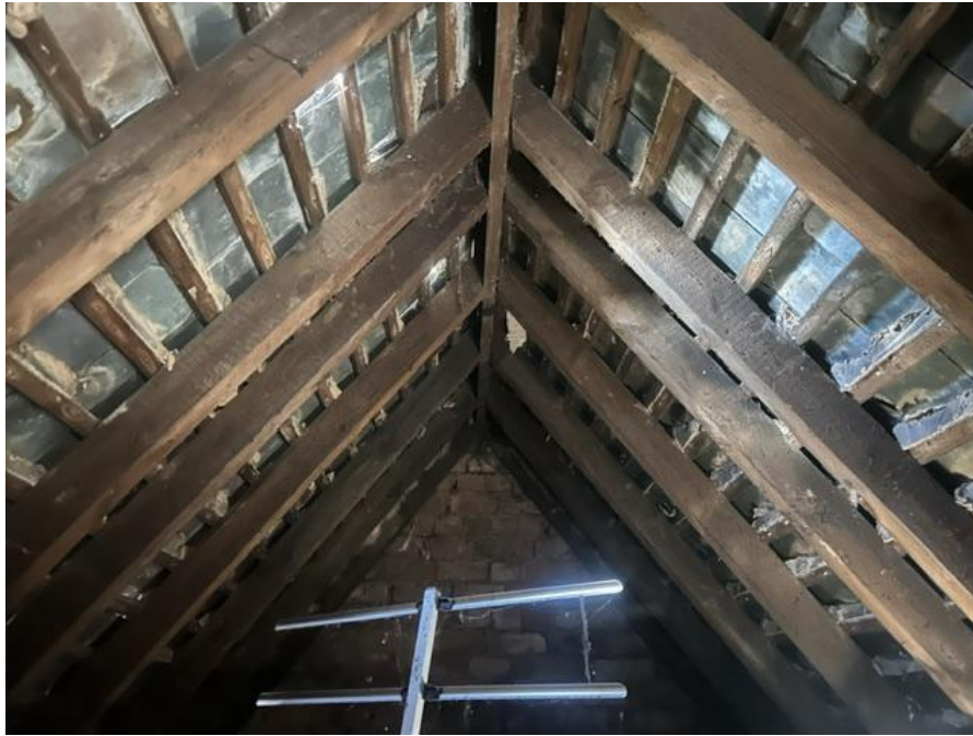
Figure 10 – Internal loft space B1
