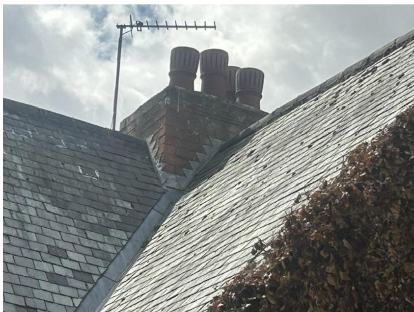
Figure 4 – View of the roof of B1
