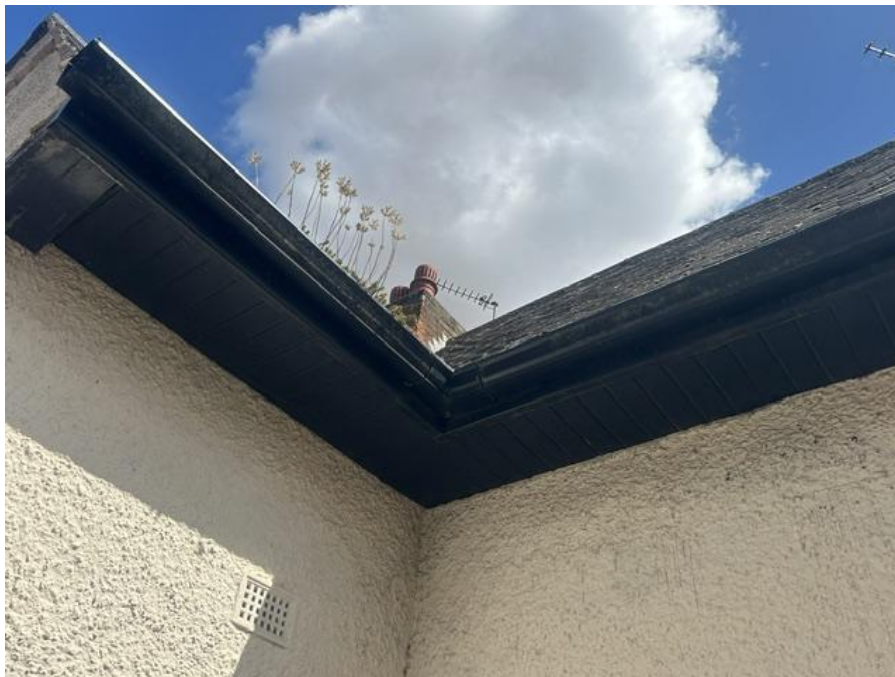
Figure 9 – Soffits tightly sealed
