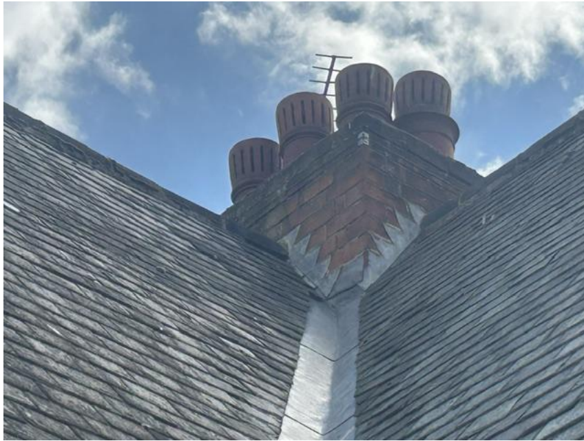
Figure 8 – Flashing tightly sealed
