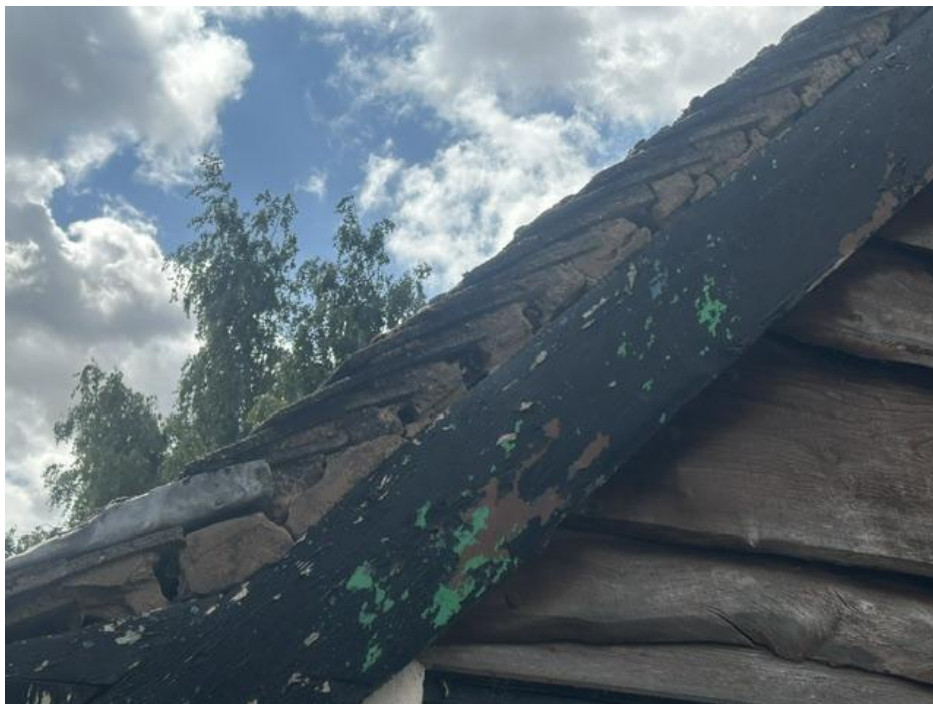
Figure 13 – Multiple gaps in bricks on B2
