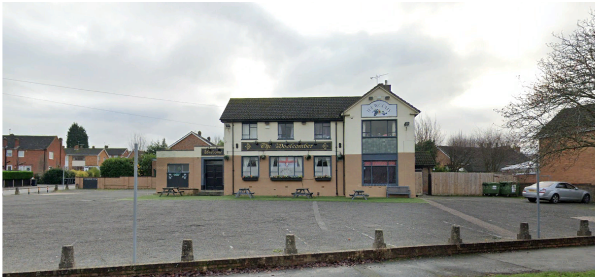
The Woolcomber — existing building
