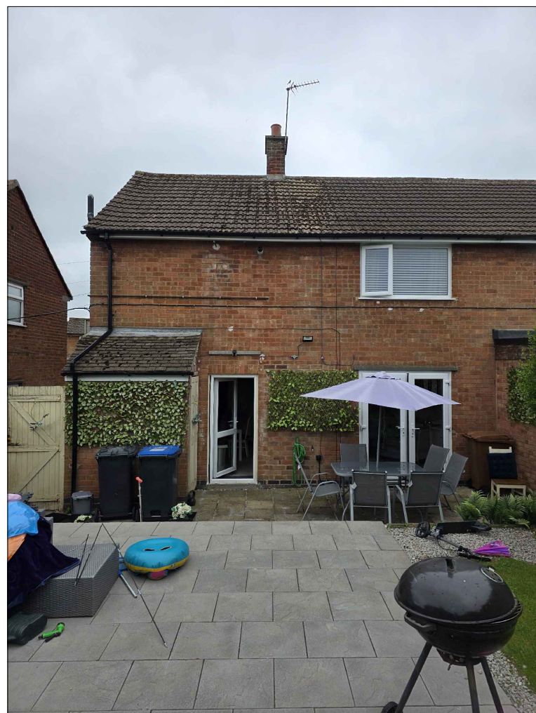
Photo of Rear Elevation
