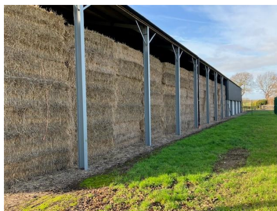
Fig 3: Northern elevation of Building 4
