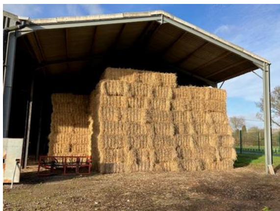
Fig 2: Eastern elevation of Building 4
