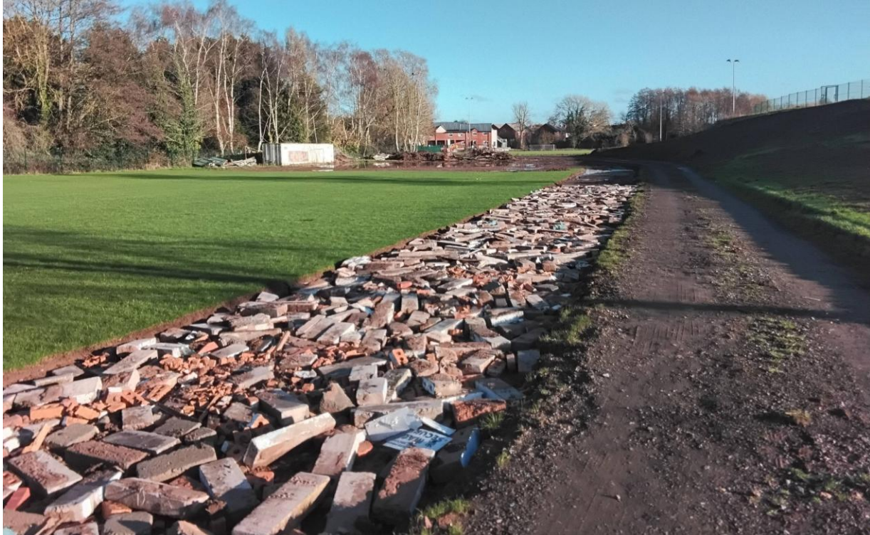
Photo 4: Area dug out and filled with rubble and bricks (photo facing northeast)
