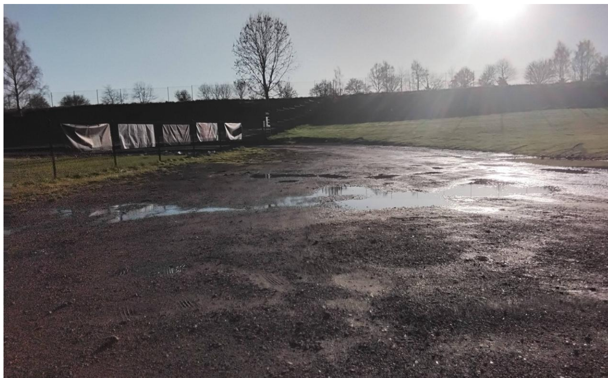
Photo 9: Area of unsealed surface near Site entrance (photo facing south).
