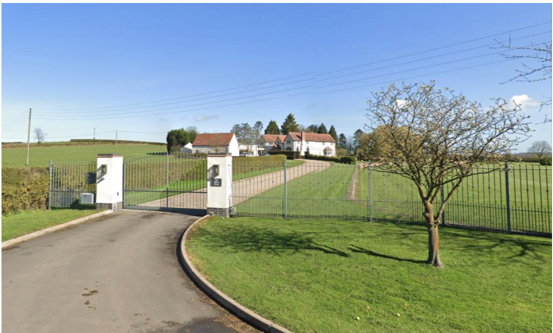
Figure 7.0.2 97 Bosworth Road, Wellsborough, Nuneaton, CV13 6PB
