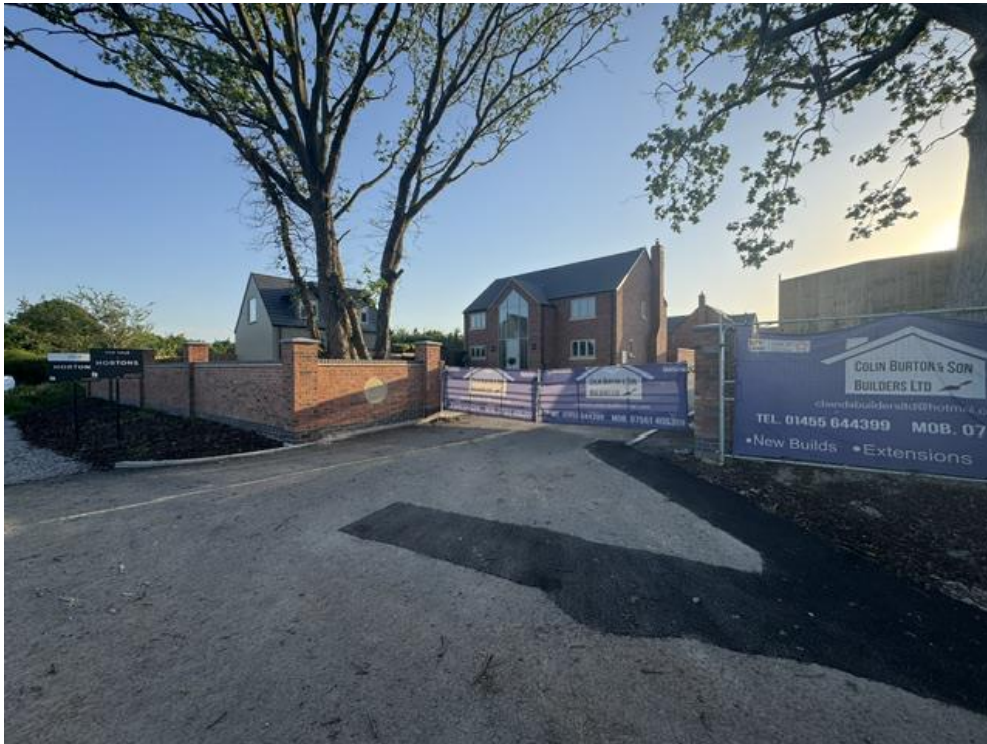
Figure 7.0.5 Adjacent street scene to appeal site [Breach Lane, Earl Shilton, LE9 7FB]
