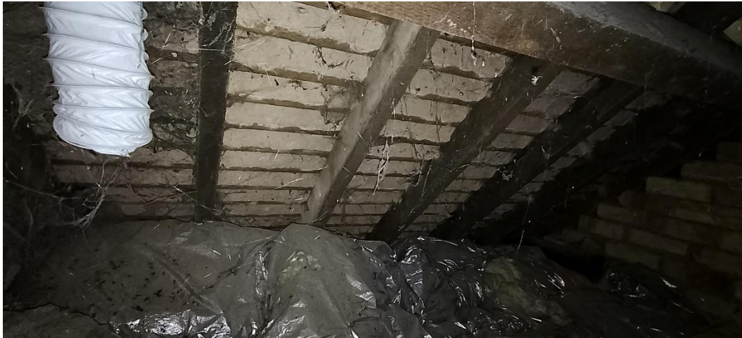
Photograph 1: Internal view of roof void.
