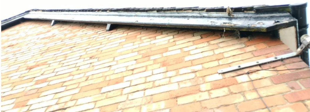
Photograph 10: View of fascias on external elevation.
