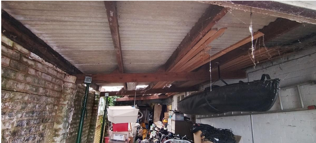
Photograph 5: Internal roof structure with exposed timbers.
