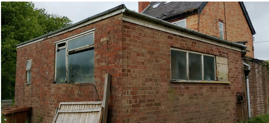
Photograph 4: External view of single-storey outbuilding.
