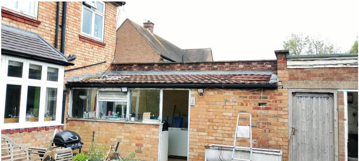
Photograph 12: Rear elevation showing lean-to extension and roof covering.
