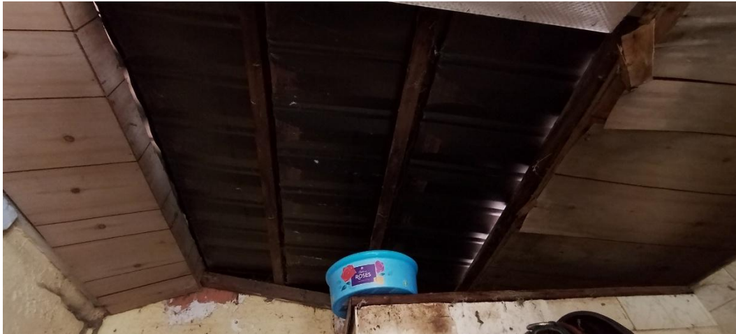
Photograph 7: Internal roof structure.
