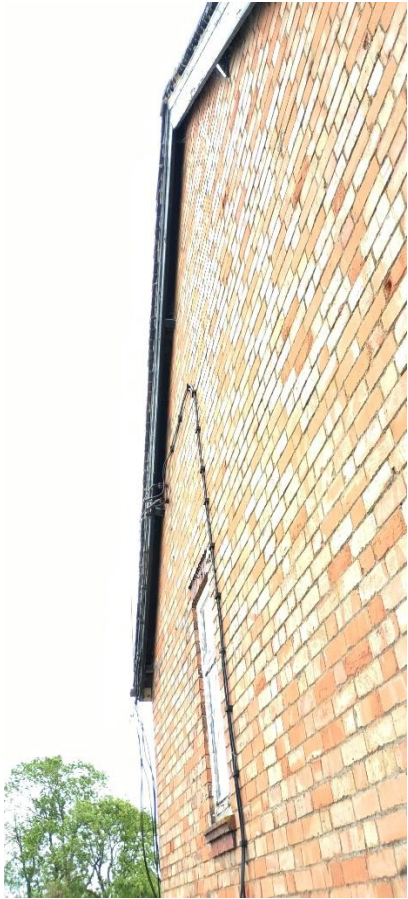
Photograph 9: View of fascias on external elevation.
