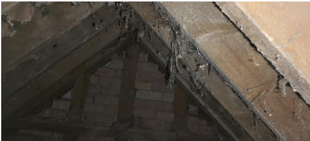
Photograph 2: Internal view of roof void.
