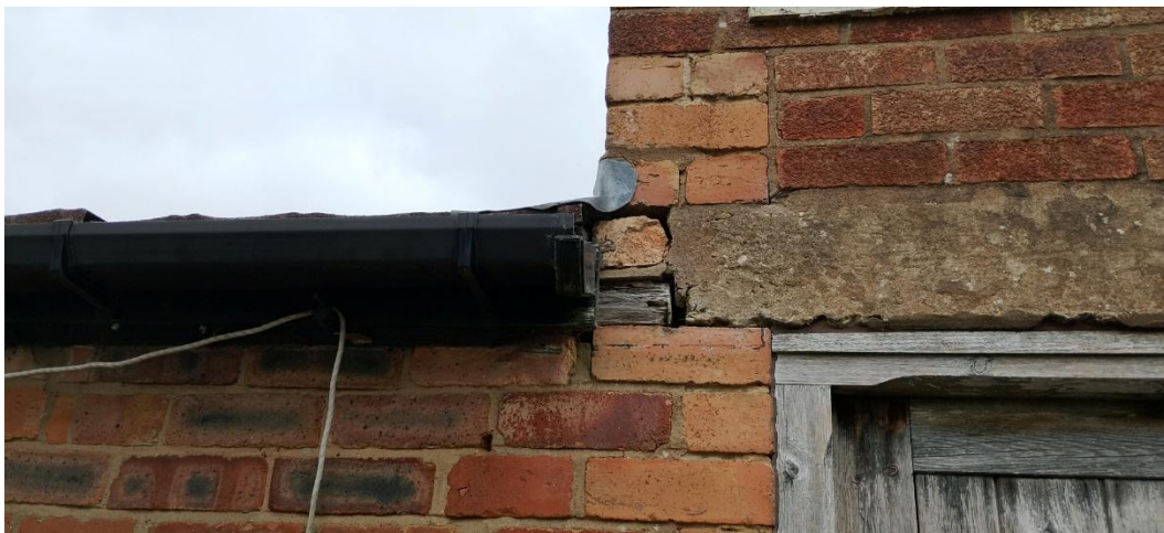
Photograph 8: Close-up of brickwork.
