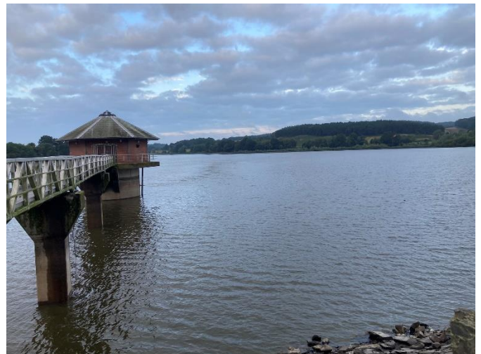
Figure 10: Looking west from Reservoir Road at eastern end of Cropston Reservoir
