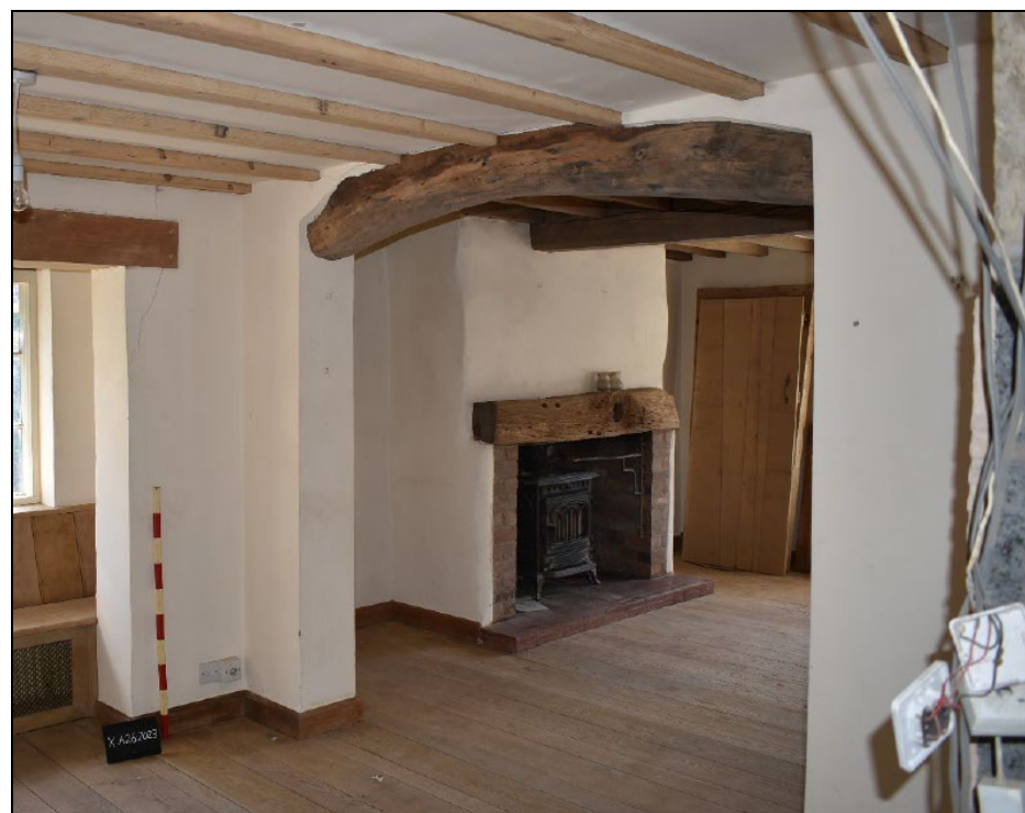
Plate 21: GF04 looking SSE into GF12 (1.0m scale)
