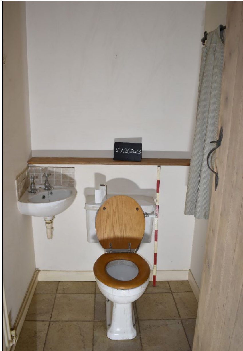
Plate 23: GF06 looking WNW (1.0m scale)
