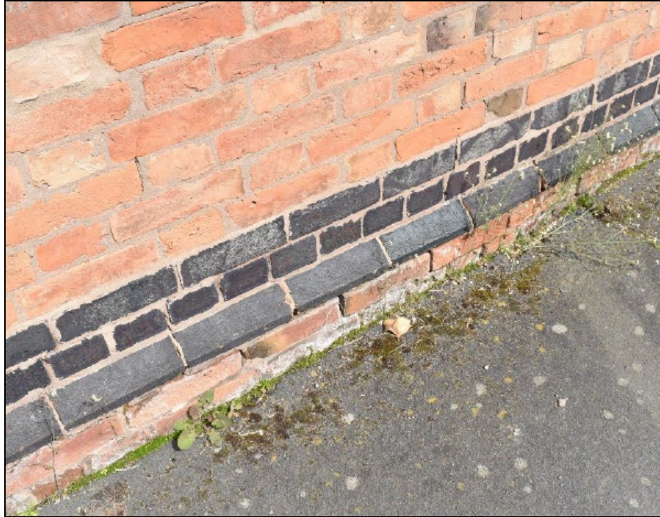
Plate 9: South elevation low blue and red brick plinth
