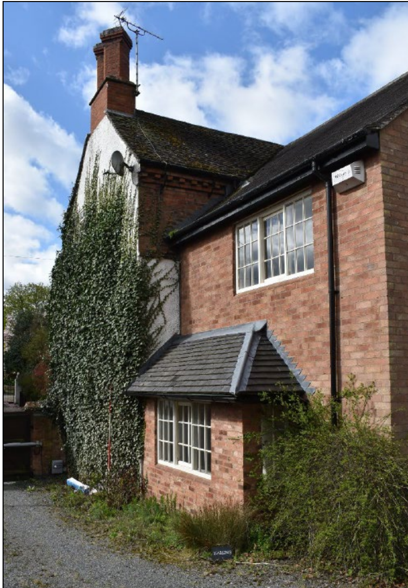
Plate 6: East elevation looking SSW (2.0m scale)
