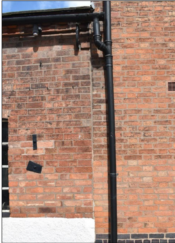
Plate 8: South elevation construction joint between Buildings A and B looking north
