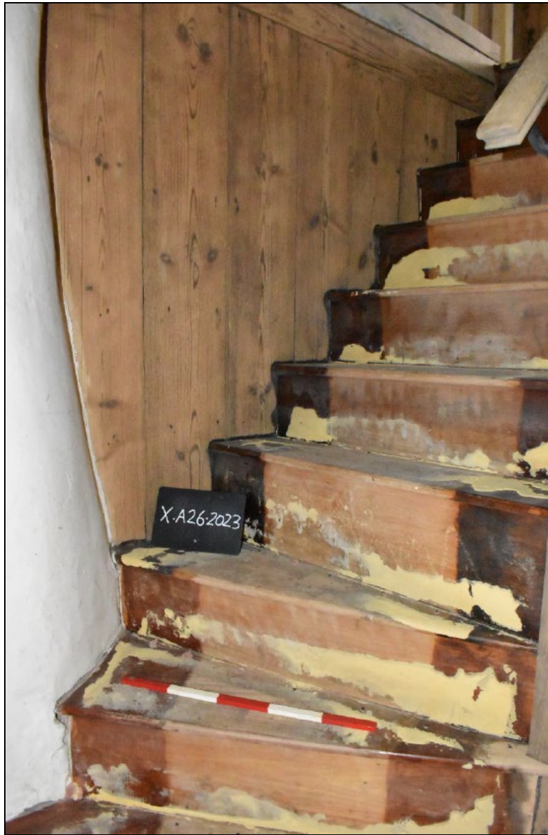
Plate 41: SF03 staircase looking WSW (50cm scale)
