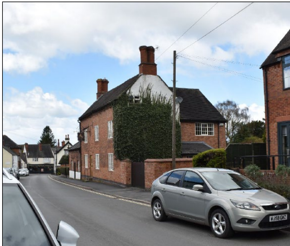
Plate 2: General view of Buildings A and B looking NW
