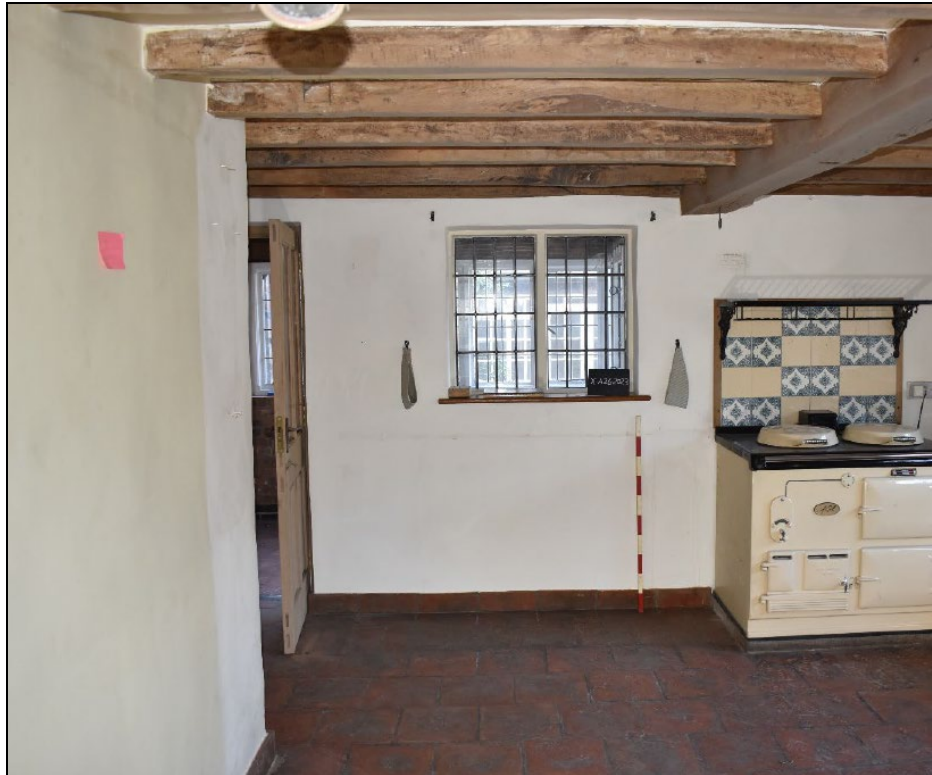
Plate 18: GF02 looking WNW (1.0m scale)
