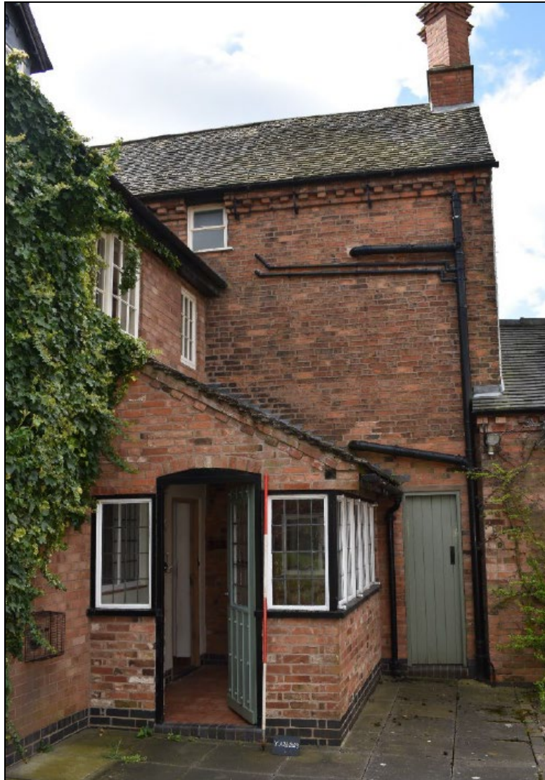
Plate 4: Porch GF01 looking south (2.0m scale)
