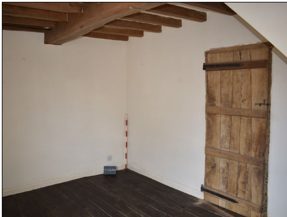
Plate 38: FF04 looking NW (1.0m scale)
