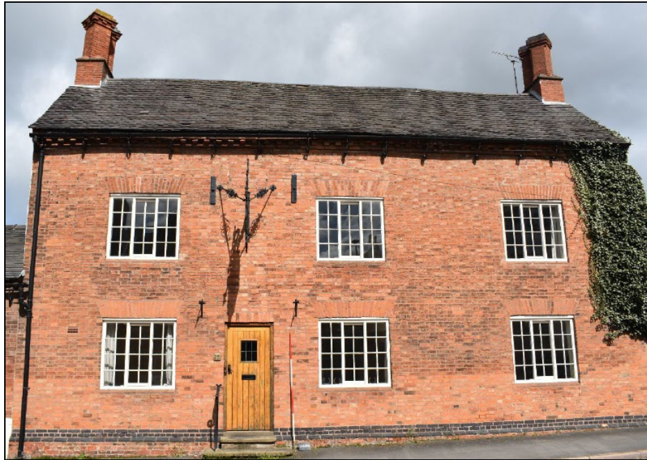
Plate 3: South elevation looking north (2.0m scale)
