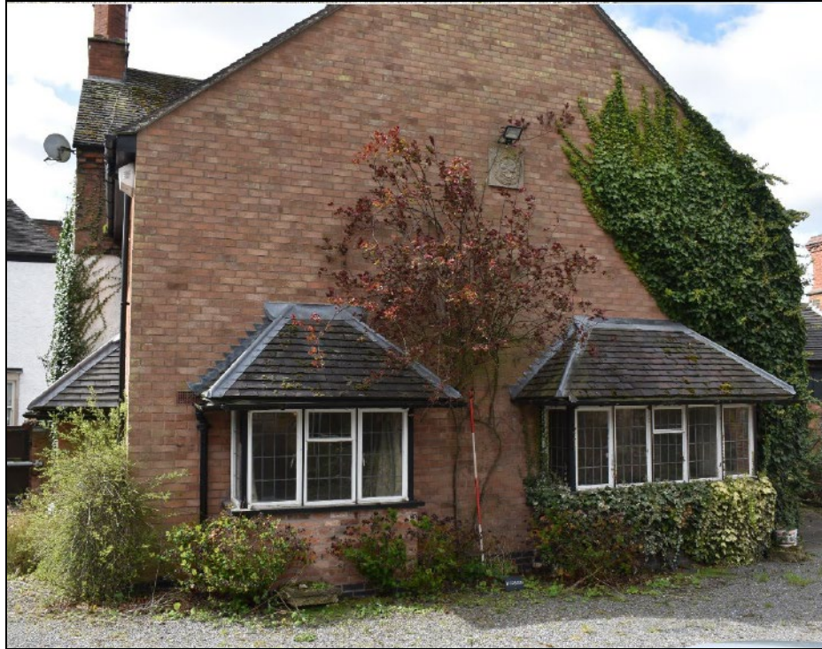
Plate 5: North elevation looking SSW (2.0m scale)
