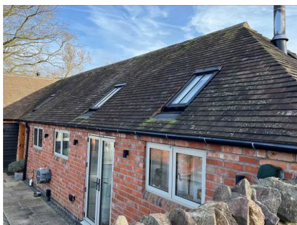
West facing roof structure
