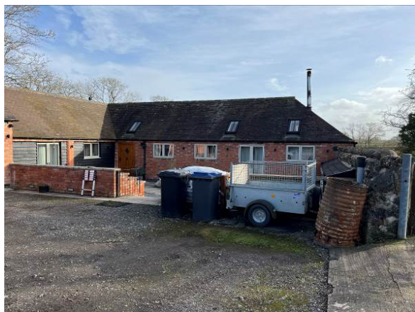
Front (west face) and yard
