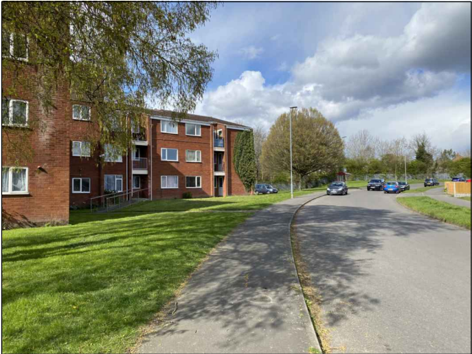
View from Astley Road to Flat 9 - 20
