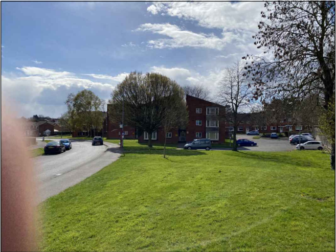
View down Astley Road to Flats and parking area
