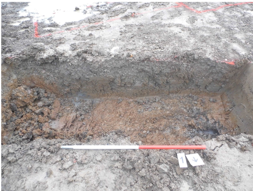
Figure 6: Foundation pit 1 looking south-west
