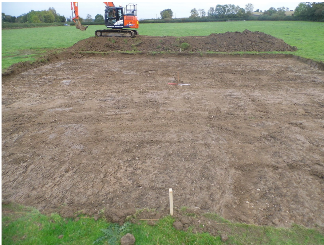
Figure 5: Stripped area looking north-east
