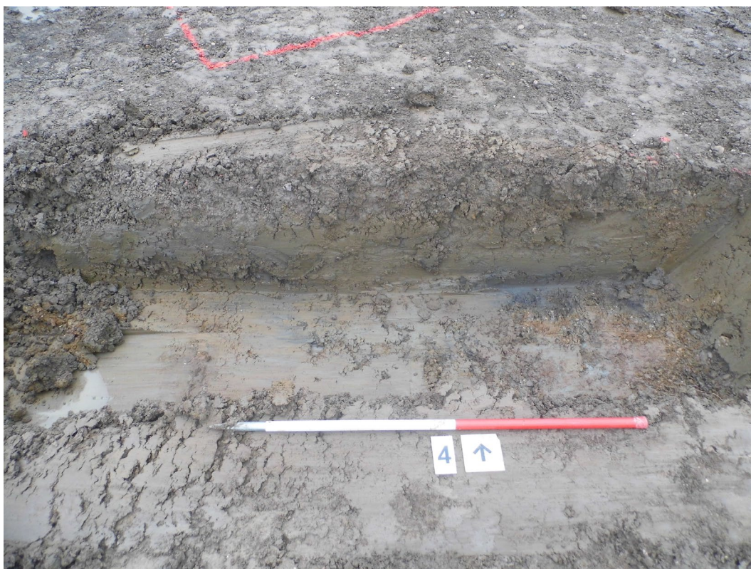
Figure 10: Foundation pit 4 looking north
