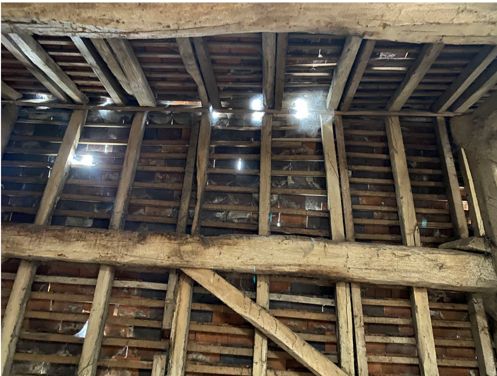
Plate 4 Building 1-Upper Level Roof
