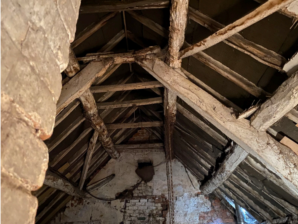
Plate 3 Building 1-Upper Level
