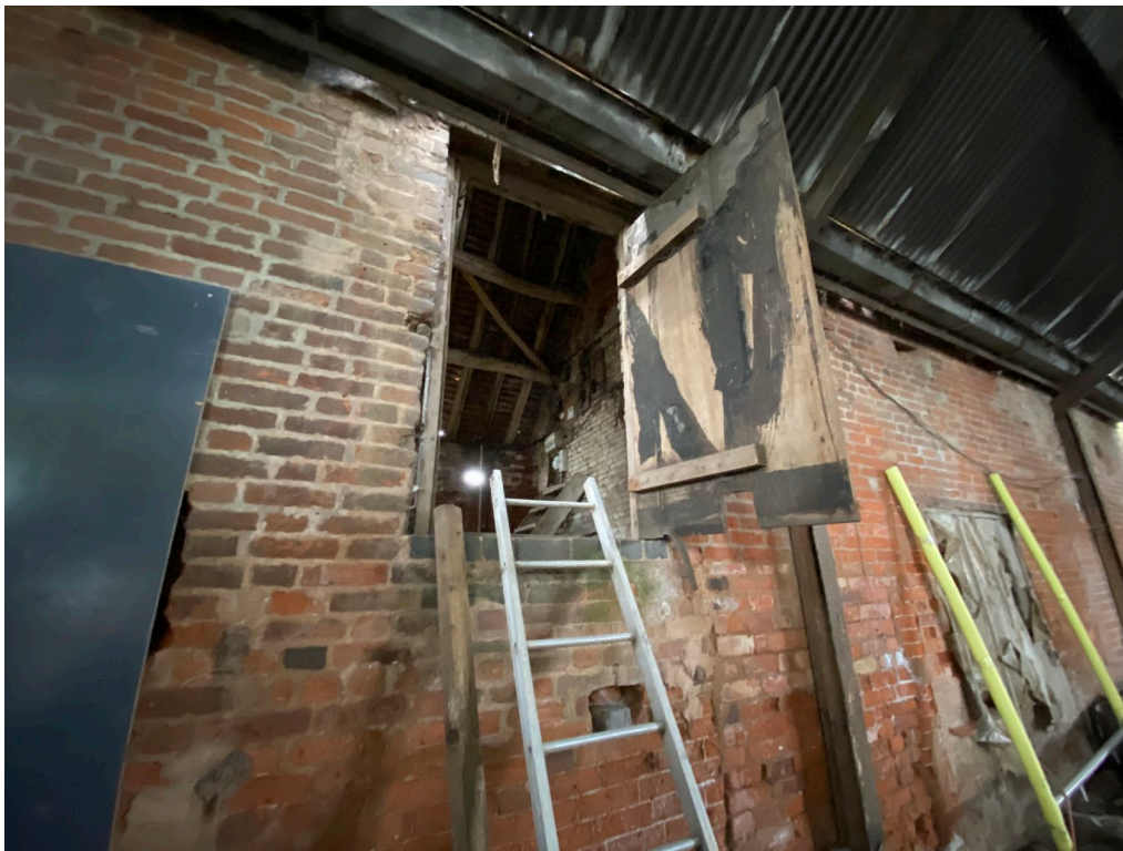
Plate 2 Building 1-Access to the Upper Level
