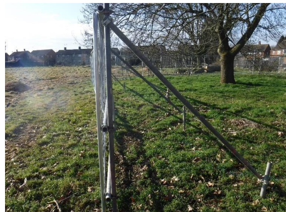
Photo 6: Scaffold driven into ground
