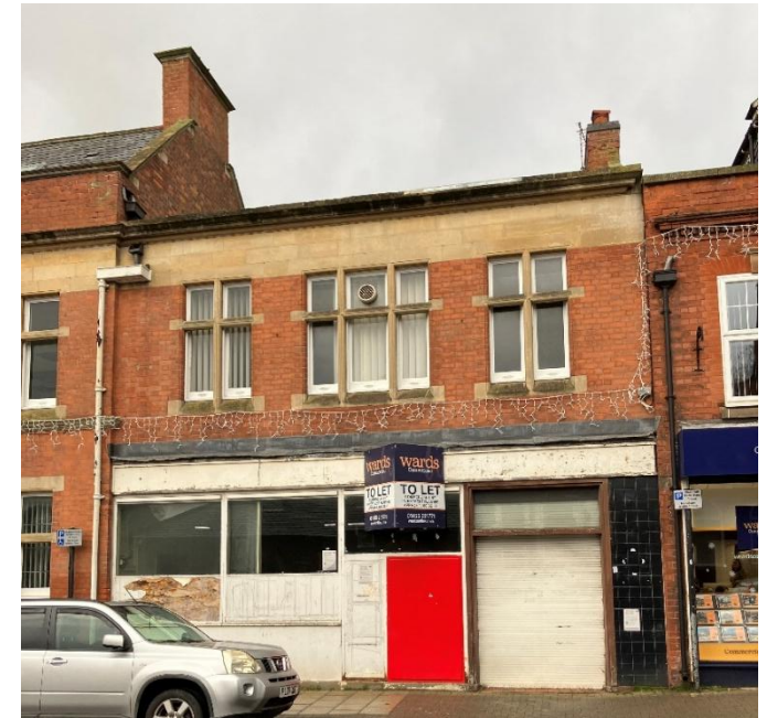
The post office counter shopfront now
