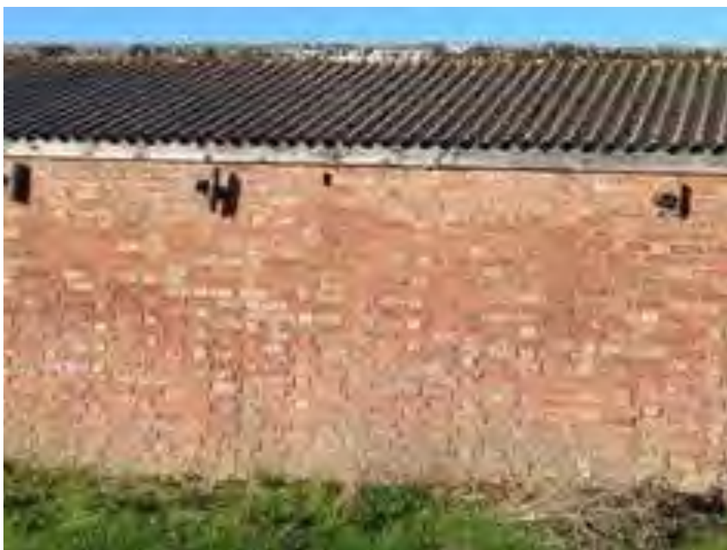
Photo 6—The majority of the barn roof.
