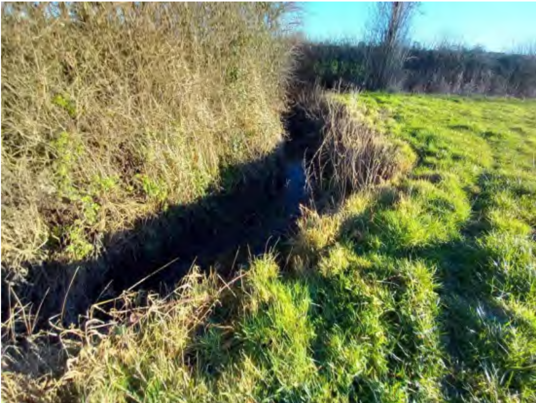
Photo 7—Tweed River at eastern boundary of site. Note high banks and overgrown brambles.
