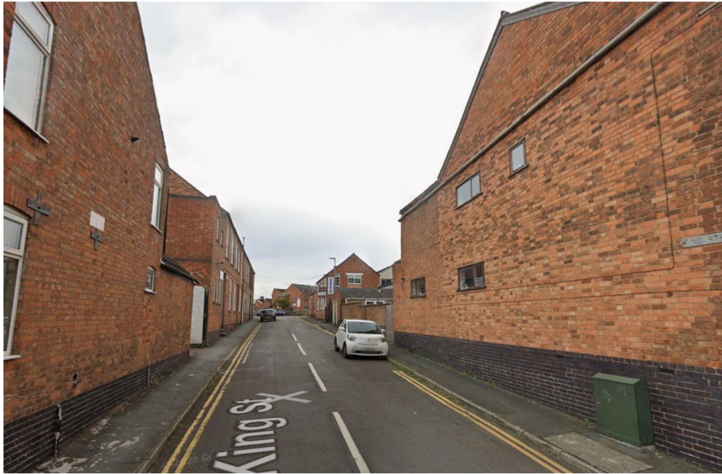
Figure 5 – The subject building on approach from the south/ Shilton Road
