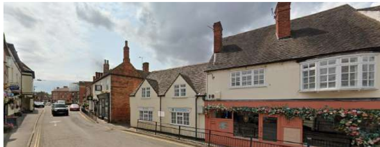
Red/orange brick, high-level render and street-facing gables
