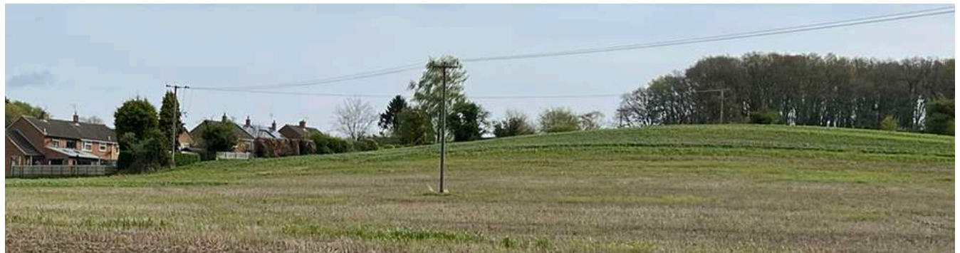
View looking north-east showing the existing overhead power lines at the eastern edge of the site
