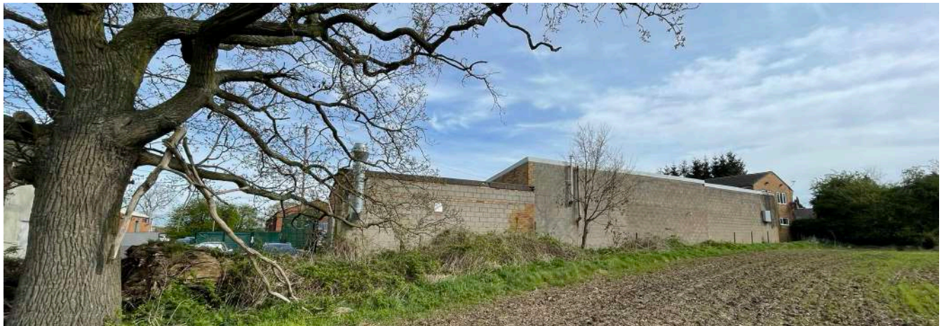
Rears of Buildings to be Demolished to form the New Site Access
