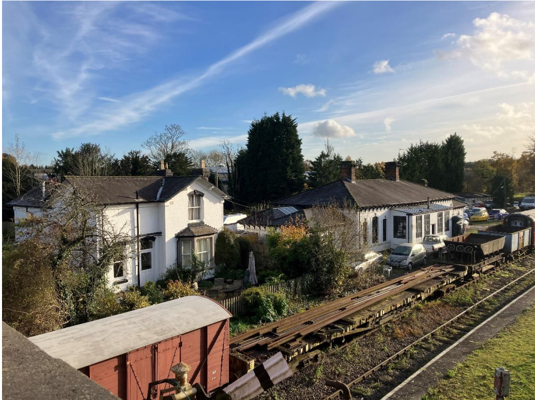
Plate 8: Station Buildings viewed from the overbridge.
