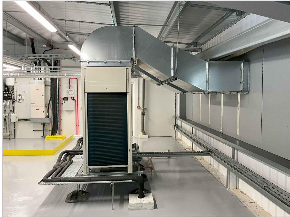
PHOTO OF EXISTING CONDENSING UNIT LAYOUT
