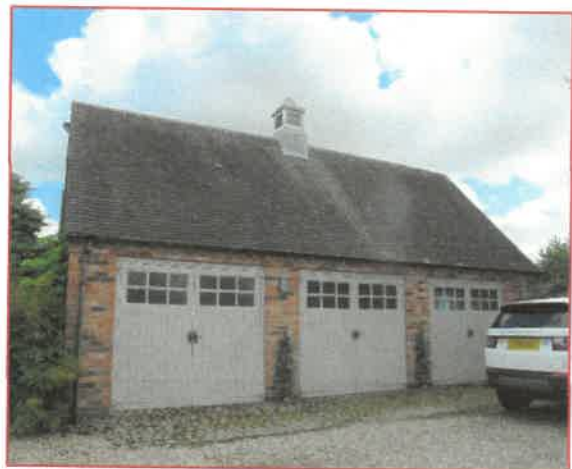
View of garage block
