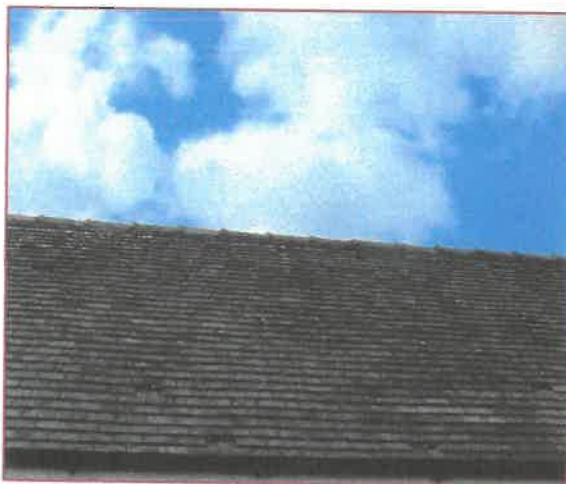
View of roof
