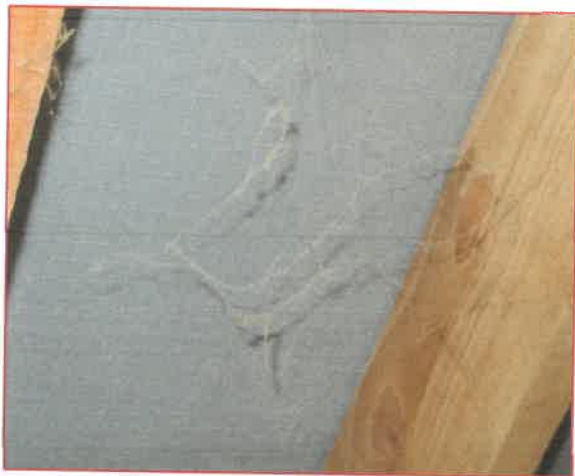
Internal view of stable block loft space
