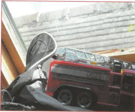
Internal view to Stable Block roof from Garage loft sky light
