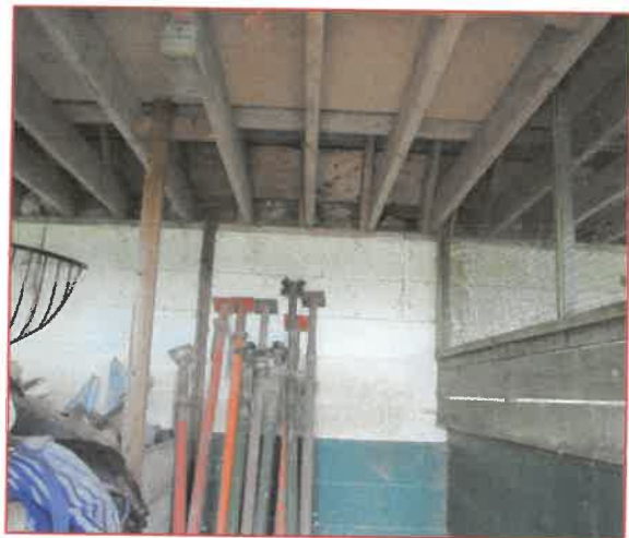
Internal view of stable block
