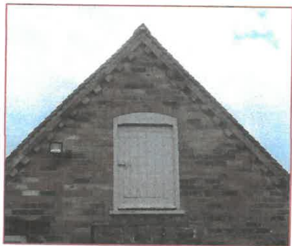
View of access door to stable block roof space
