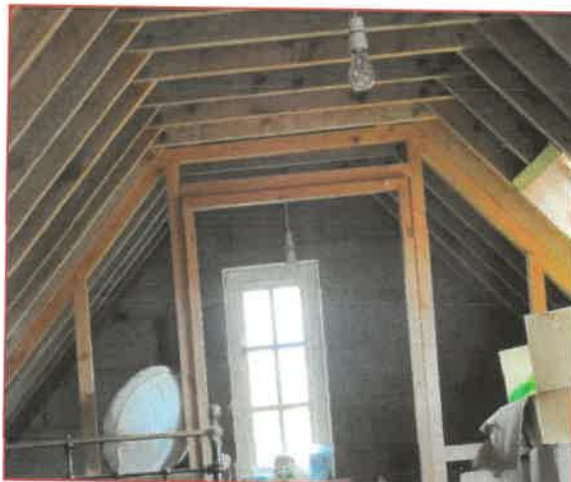
Internal view of garage roof loft
