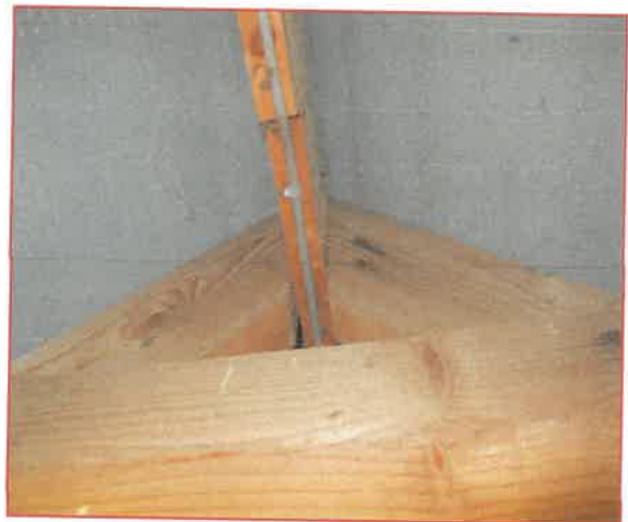
Internal view of stable block loft space
