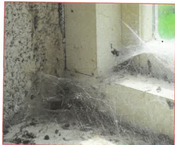
Internal view of window
