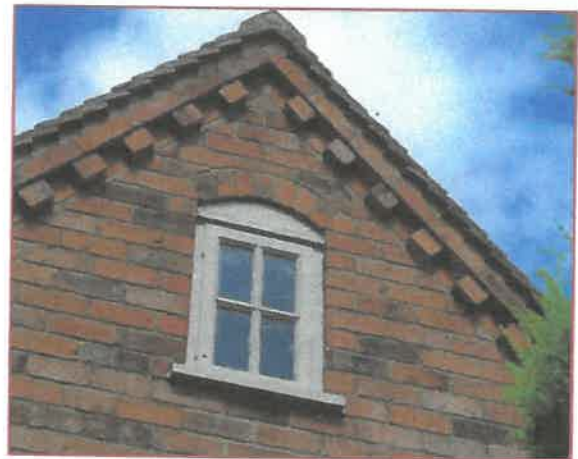
View gable end
