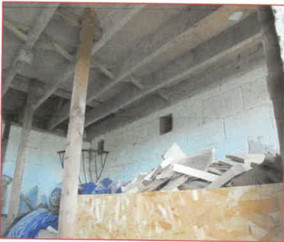
Internal view of stable block
