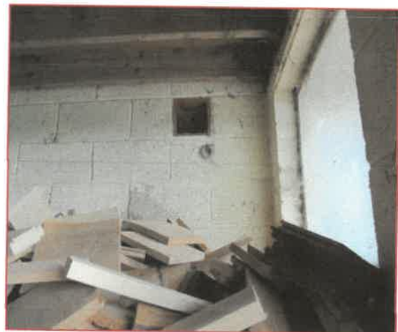
Internal view of stable block
