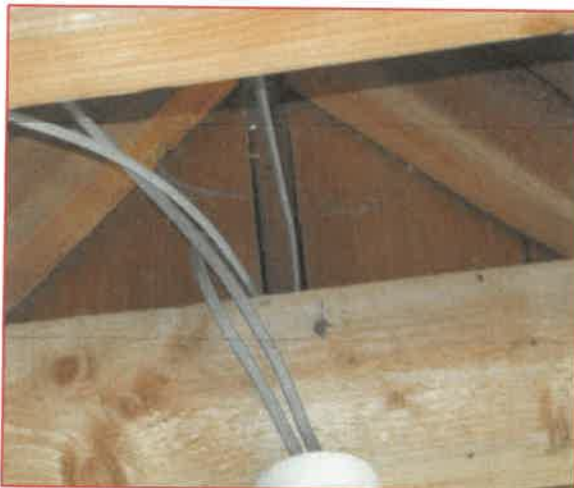
View of ridge board
