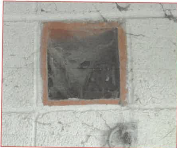
Internal view of stable block
