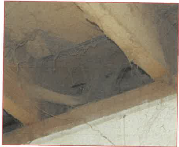
Internal view of stable block
