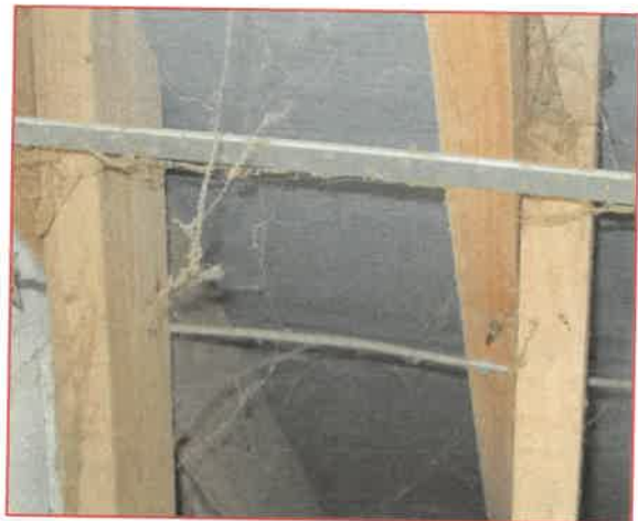
Internal view of stable block loft space
