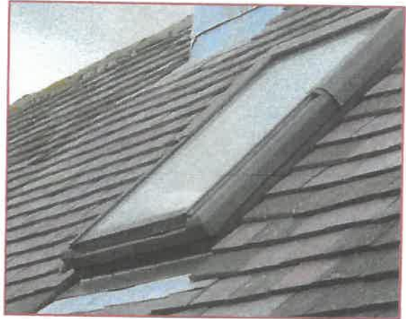
View of sky light window & lead flashing
