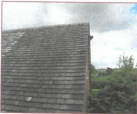
View of roof
