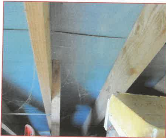
Internal view of stable block loft space
