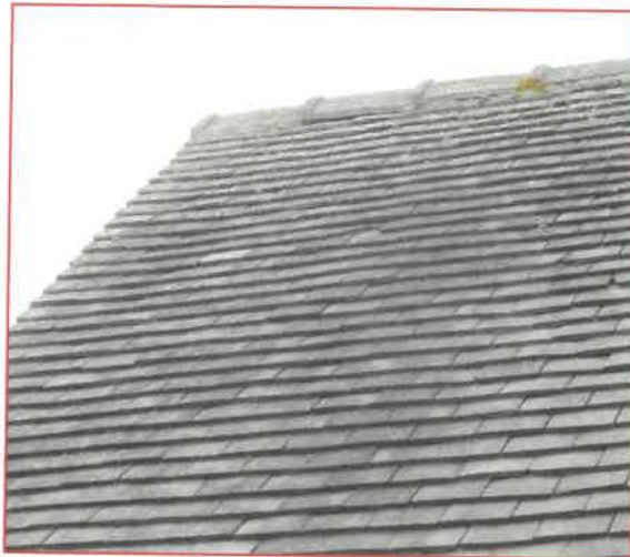
View of stable roof
