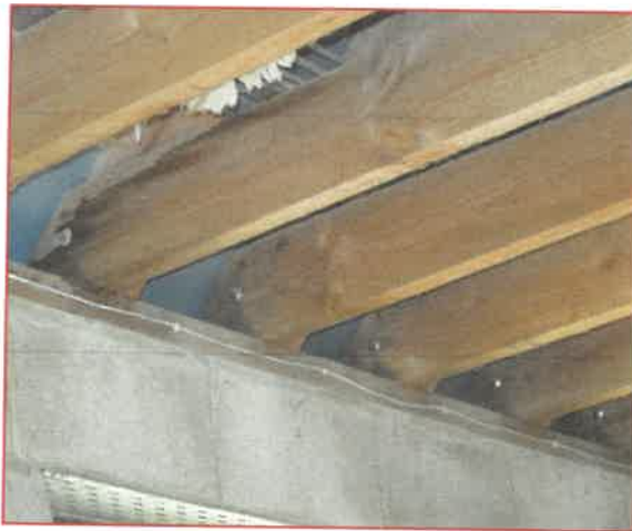
Internal view of roof & sarking felt
