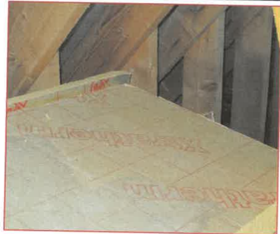
Internal view of stable block loft space
