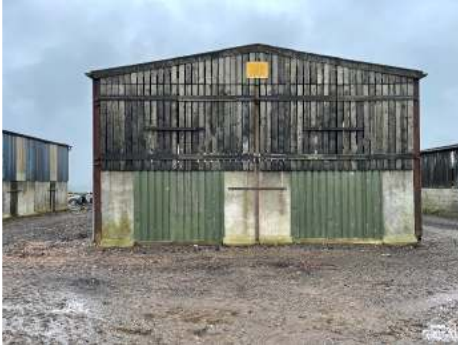
Figure 2: Barn A - rear elevation
