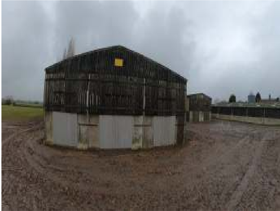
Figure 11: Barn B – Right hand side elevation
