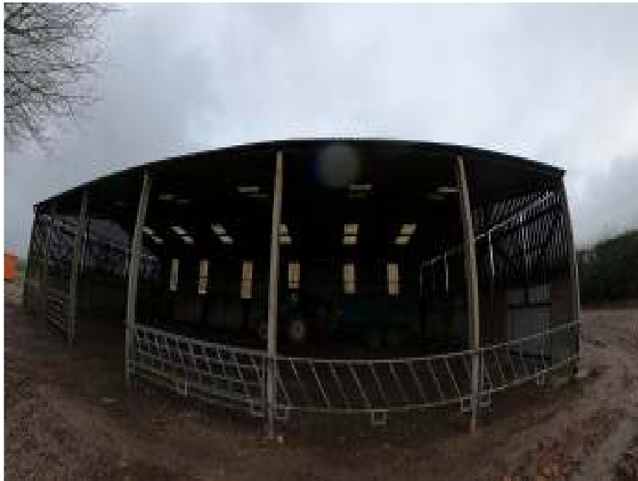
Figure 10: Barn B – Front elevation
