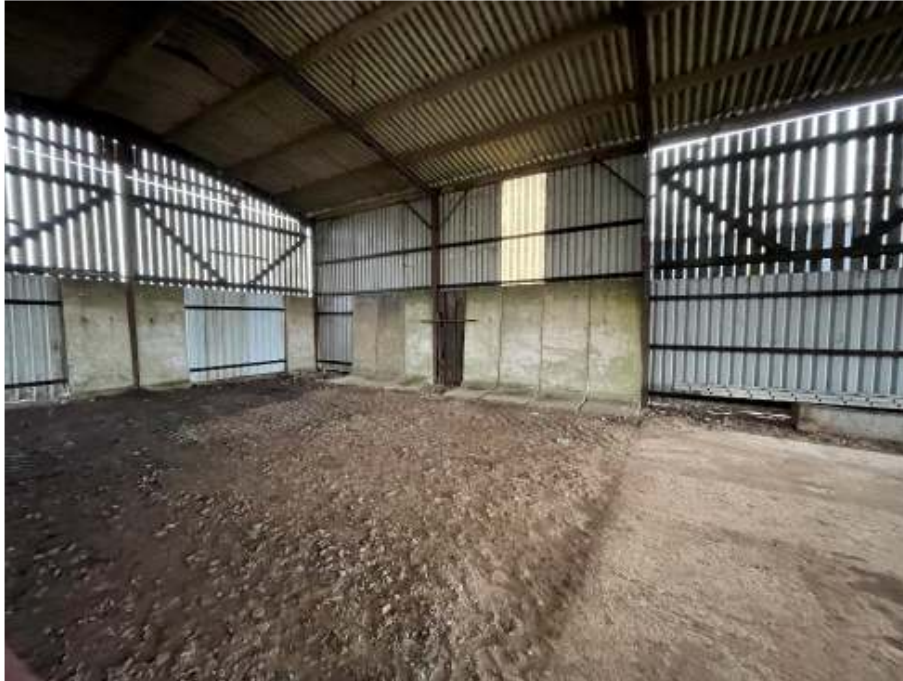
Figure 6: Barn A - knee bracing, purlins and cladding rails
