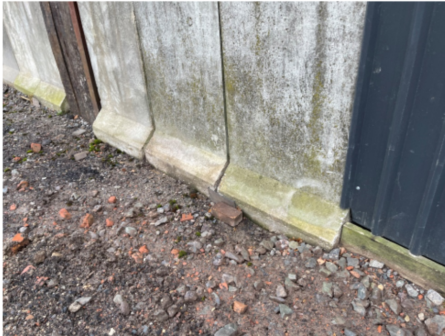
Figure 9: Barn A - precast concrete wall units
