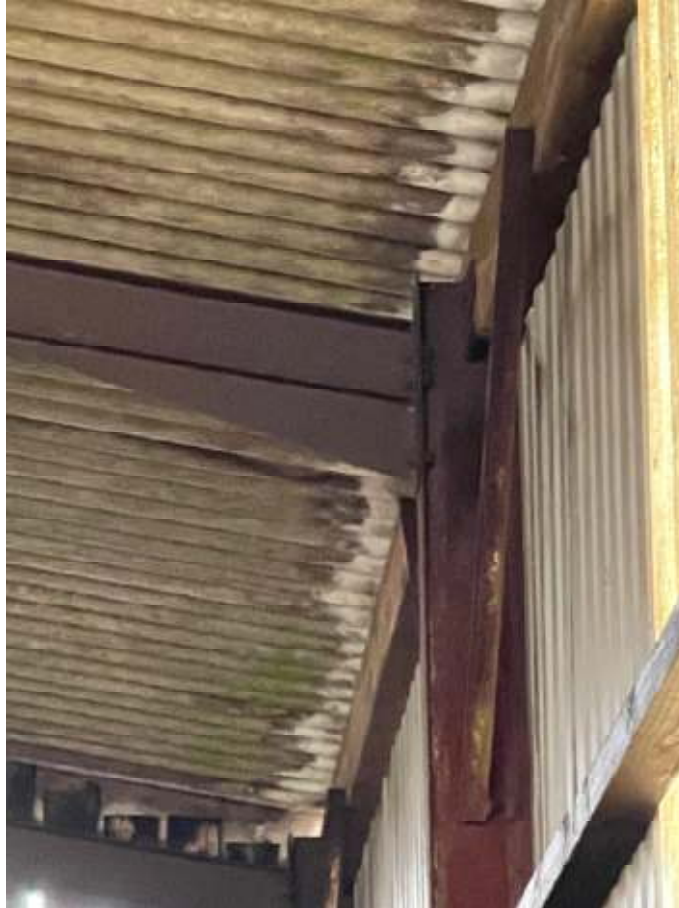
Figure 7: Barn A - portal frame eaves connection
