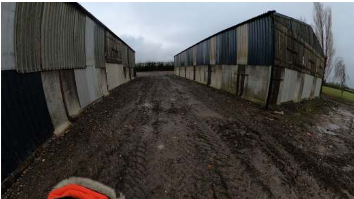
Figure 12: Barn B – Rear elevation (RHS)
