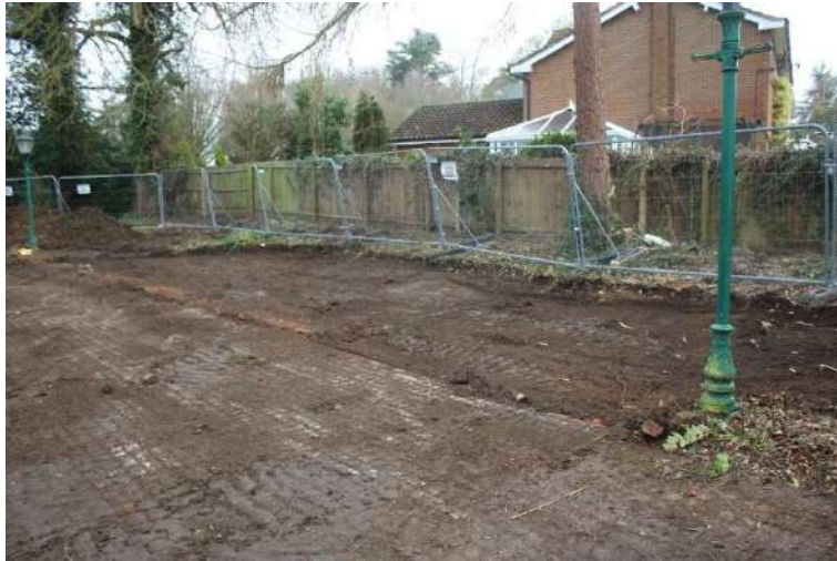
Plate 2. Area 1, west section looking northeast (no scale)
