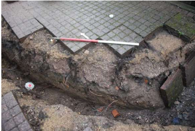
Plate 6. Southwest section of western trench for new water main, showing (109), looking northeast (1m scale)
