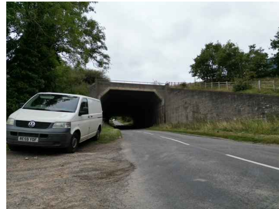
View 3. Facing left at access onto Markfield Road.
