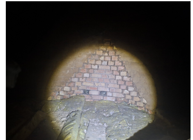
Figure 1b: B1 loft space (looking north)- floor
