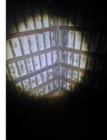
Figure 1a: B1 loft space (looking north end)
