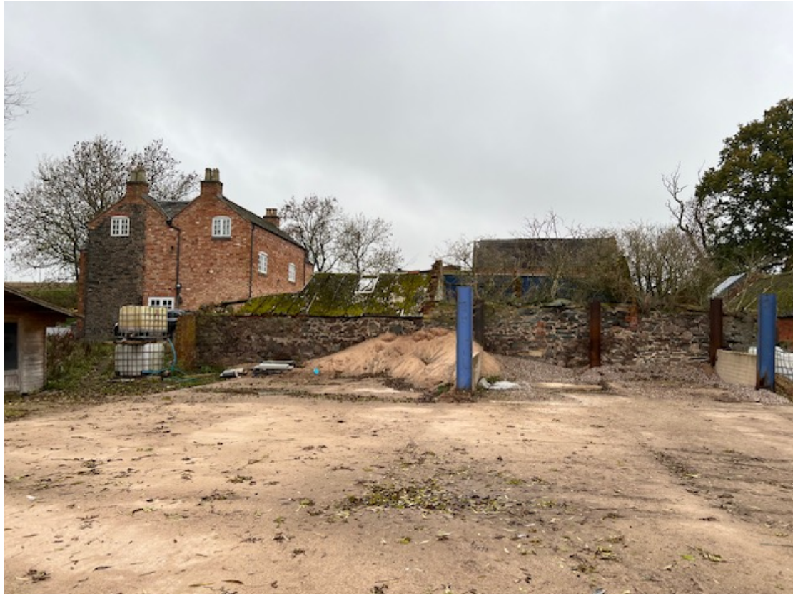
Figure 4 – Photograph showing existing concrete base and material storage
