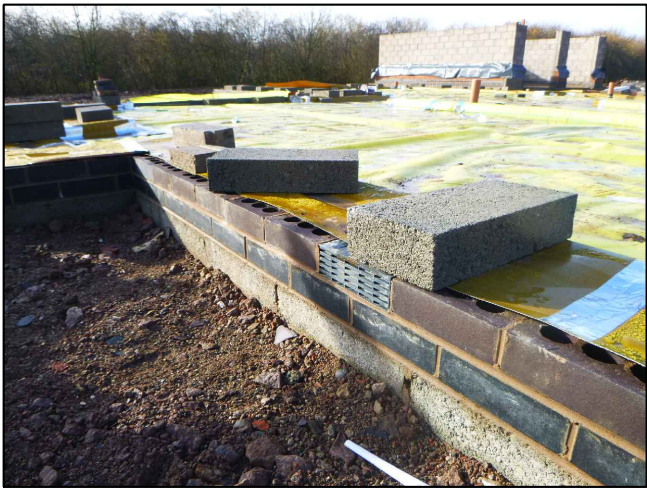
C View of Air Bricks in Plot 2
