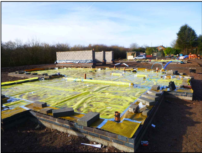
B General View of Plot 2
