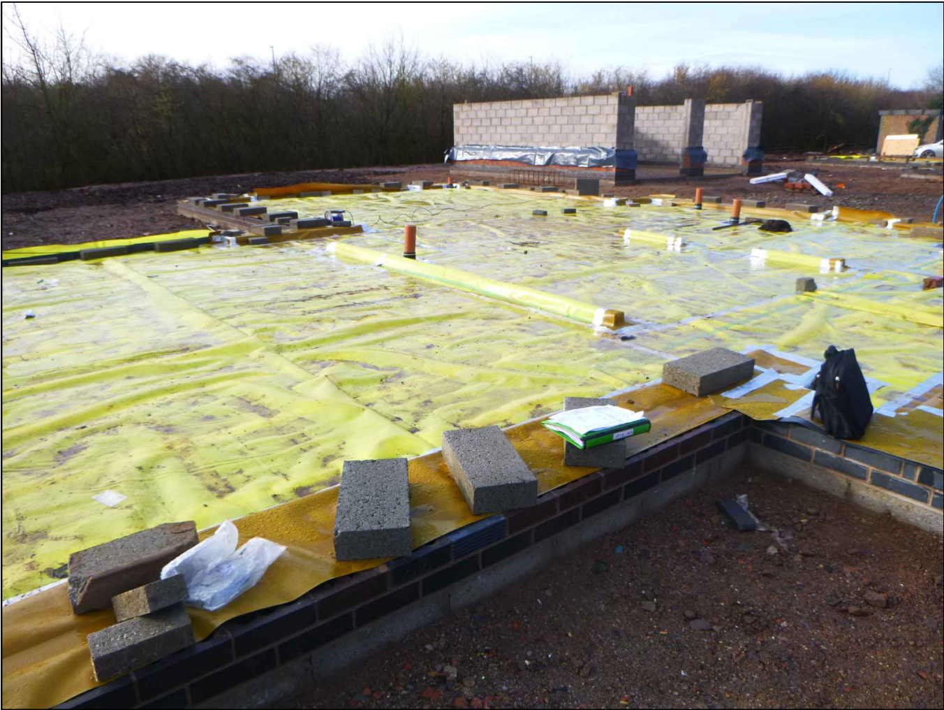
A General View of Plot 2
