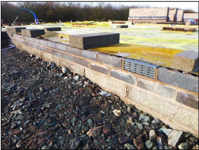
C View of Air Bricks in Plot 1
