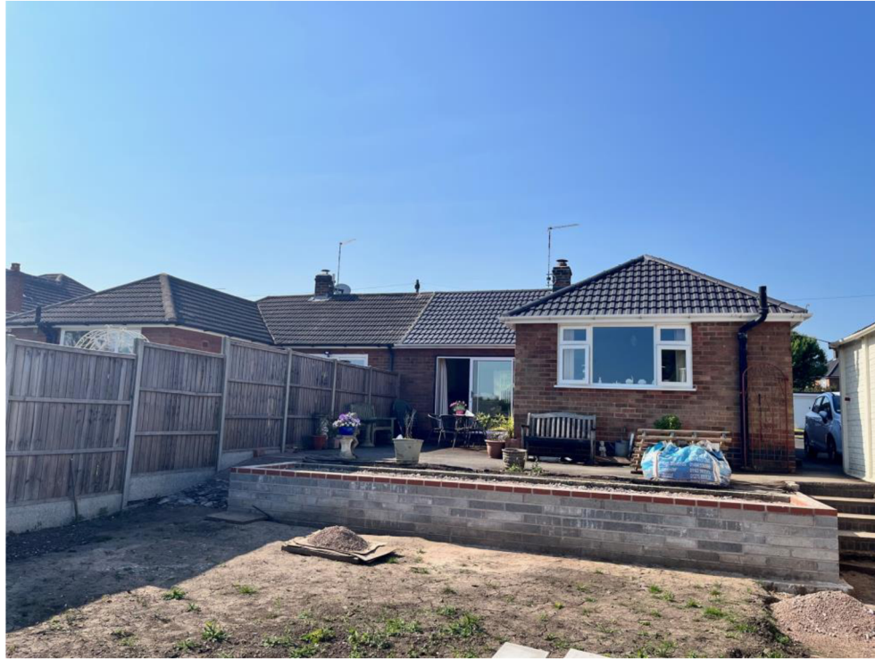
Photograph 1. The Rear Elevation
