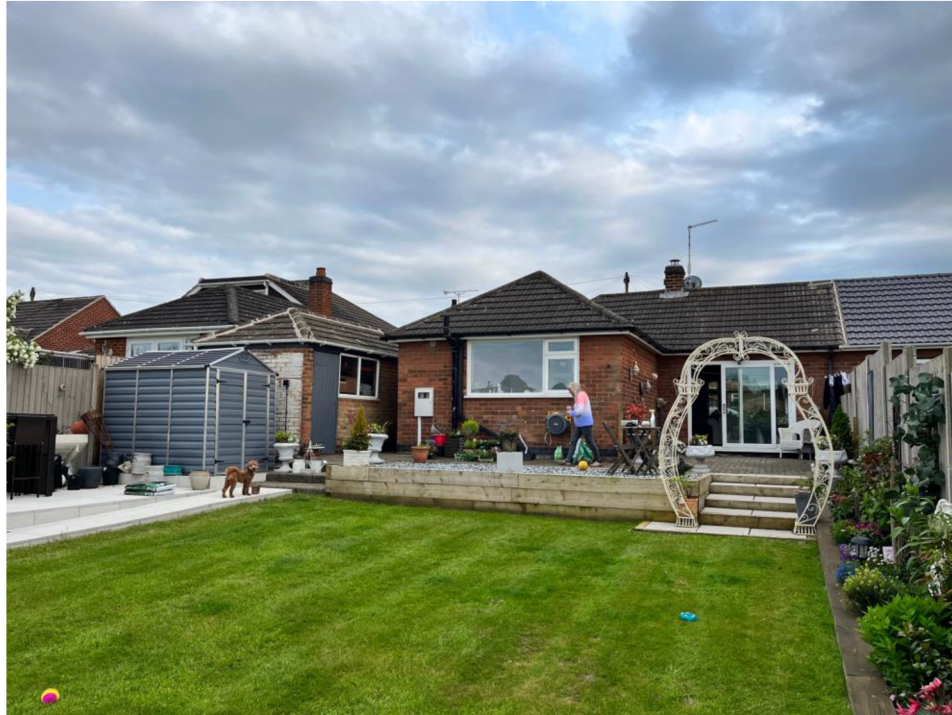
Photograph 1. The Rear Elevation
