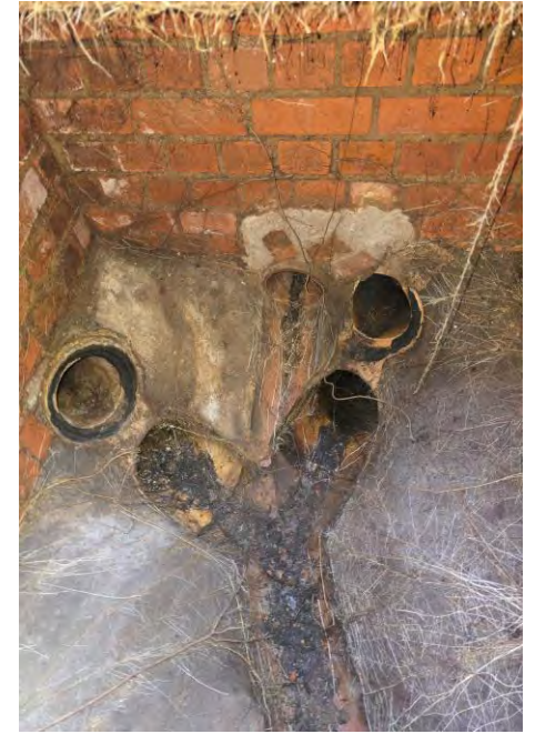
View into the proposed connection IC
