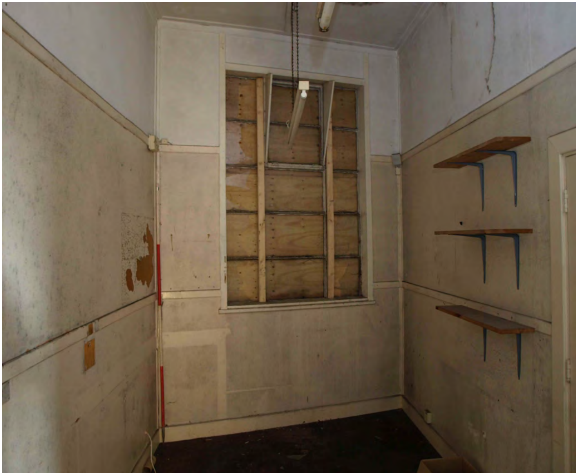
Plate 31: Office created above carriageway
