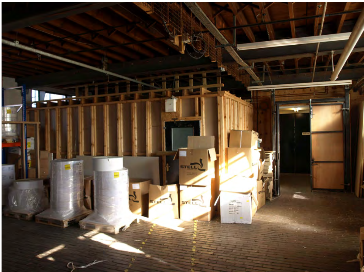
Plate 42: View looking north-east along ground floor of later extension
