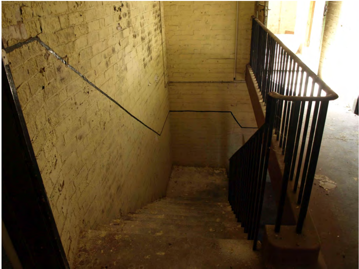
Plate 33: Stairwell looking south
