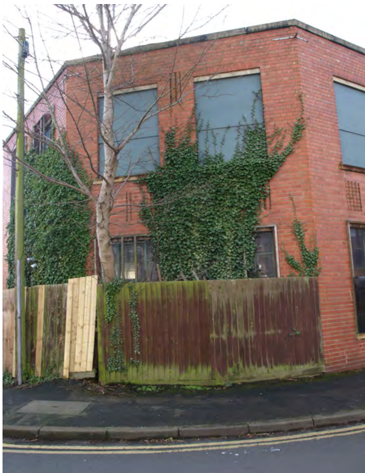
Plate 11: Eastern elevation of later extension
