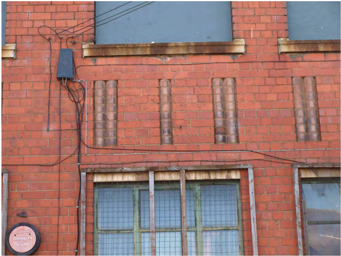
Plate 9: Detail of semicircular brick pilaster decoration
