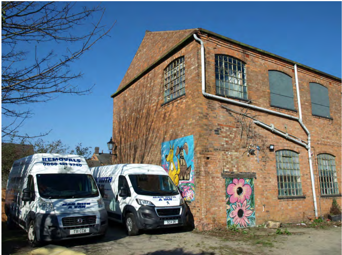
Plate 3: South facing gable end of original T shaped factory
