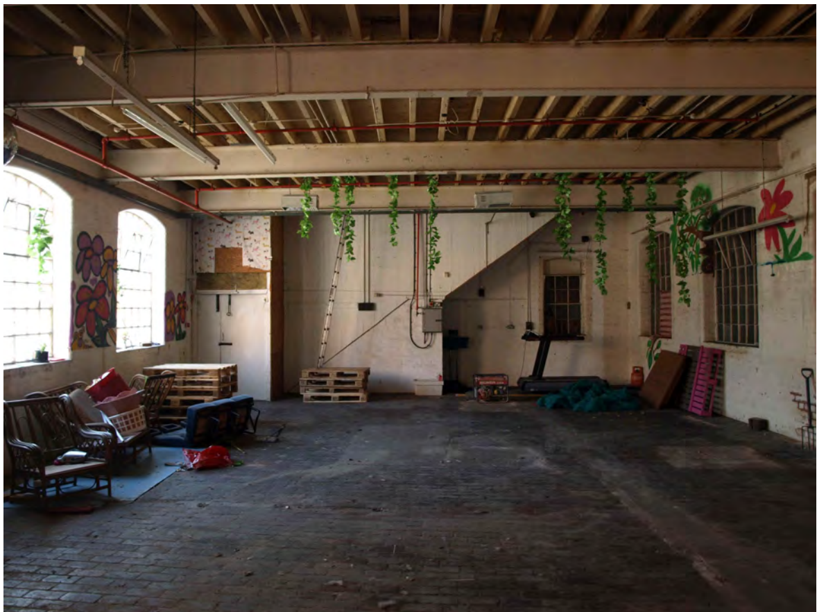
Plate 14: Southern wing of original factory looking south
