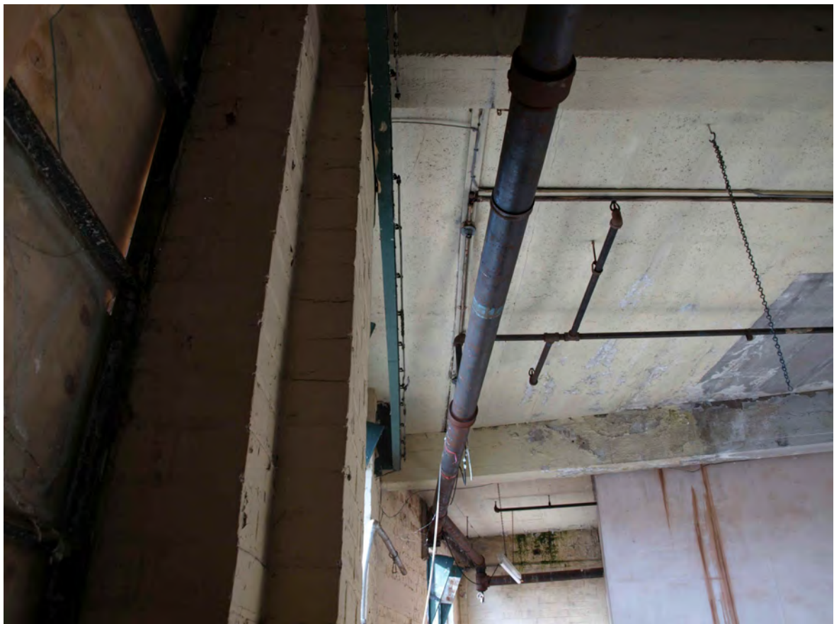
Plate 40: Detail of curtain rails to left with sprinkler system shown to right
