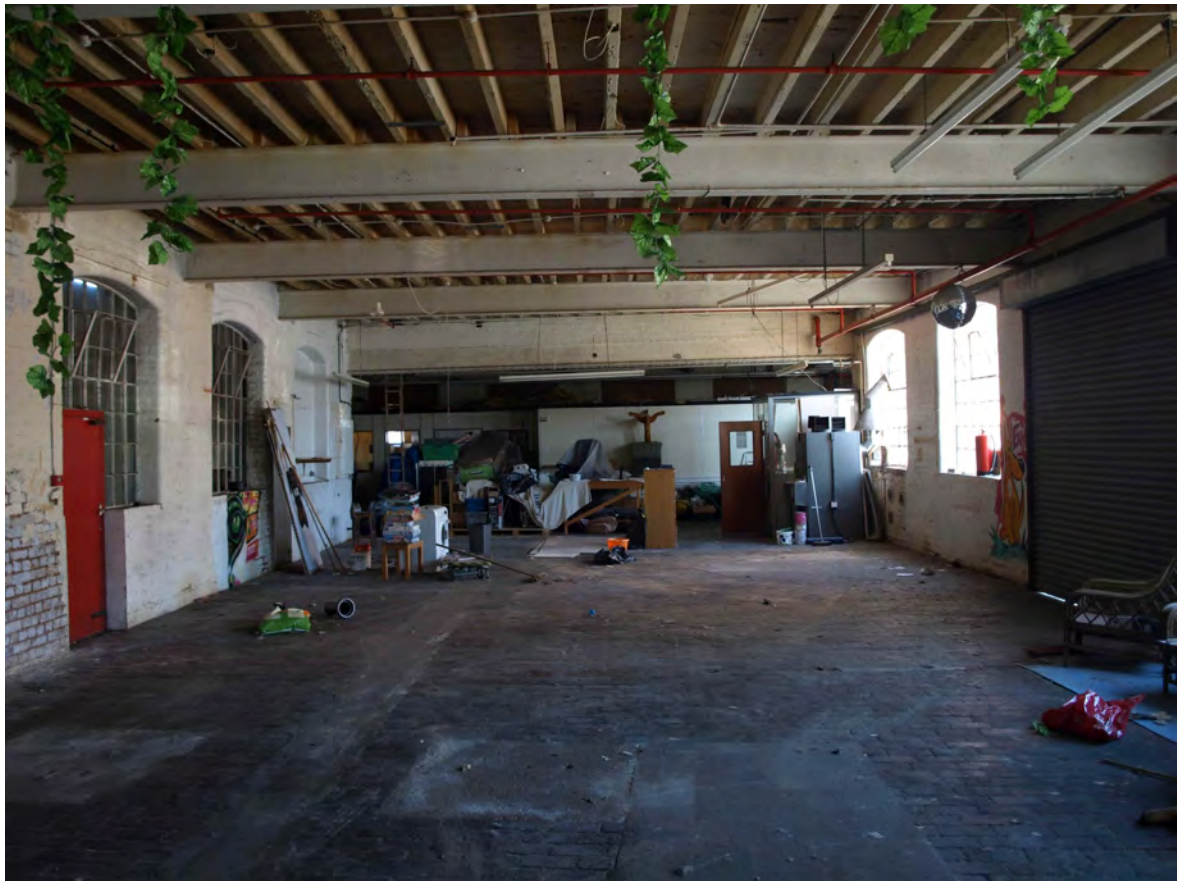
Plate 15: View of southern wing looking north towards Wood Street
