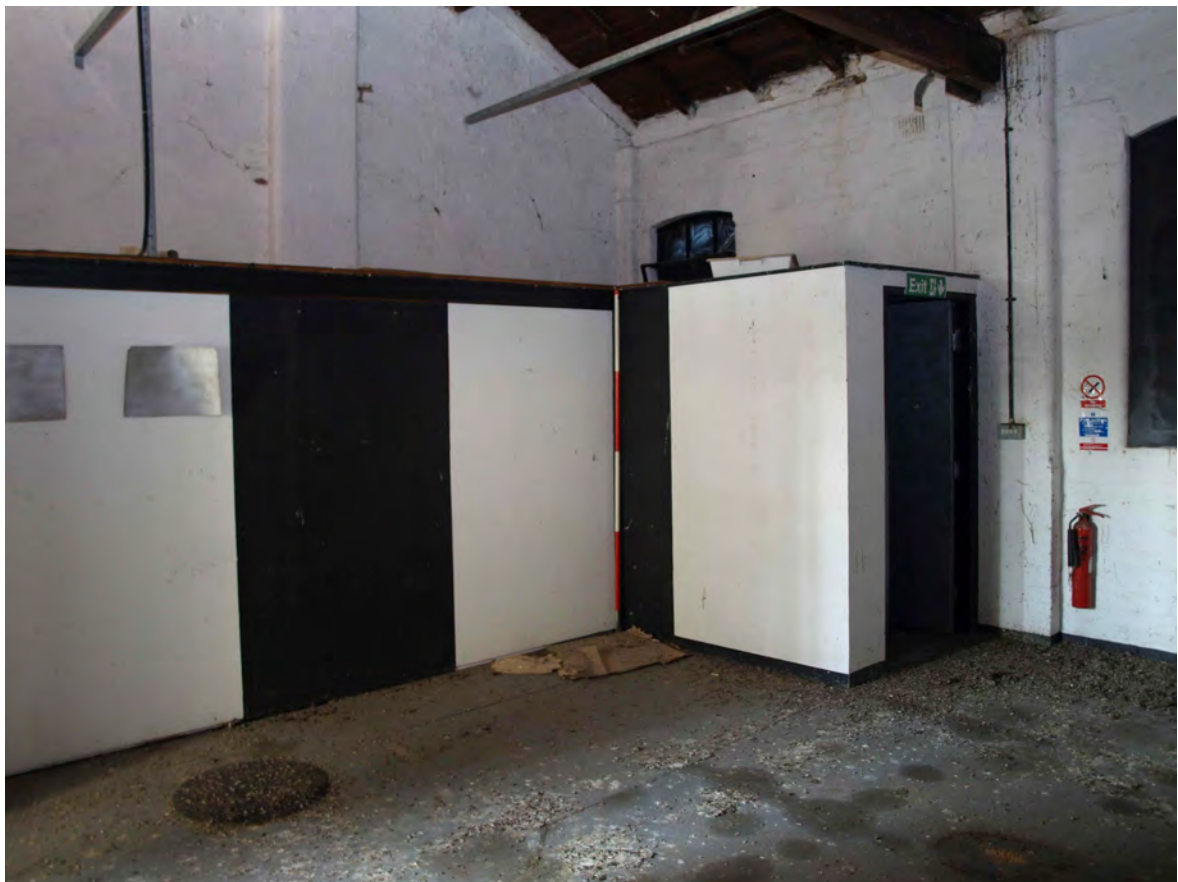
Plate 18: Later boxing in of stairwell on first floor
