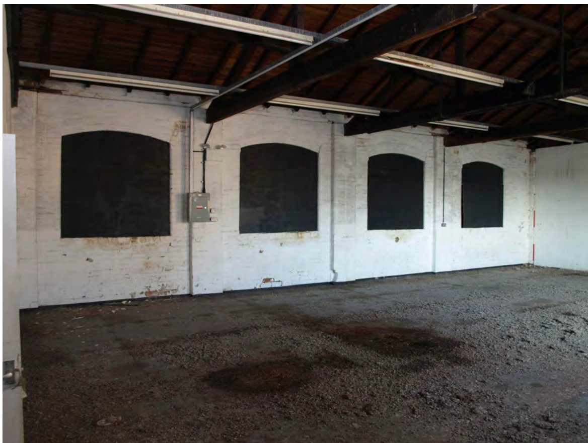
Plate 21: Internal western elevation of southern wing on first floor
