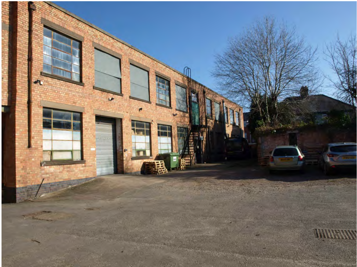
Plate 7: Southern elevation of later extension
