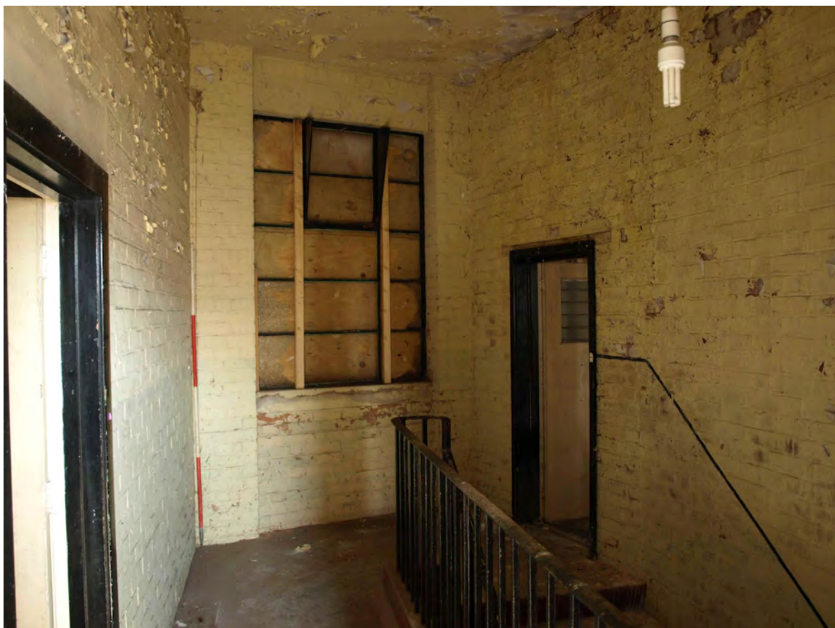
Plate 32: Stairwell looking north on first floor
