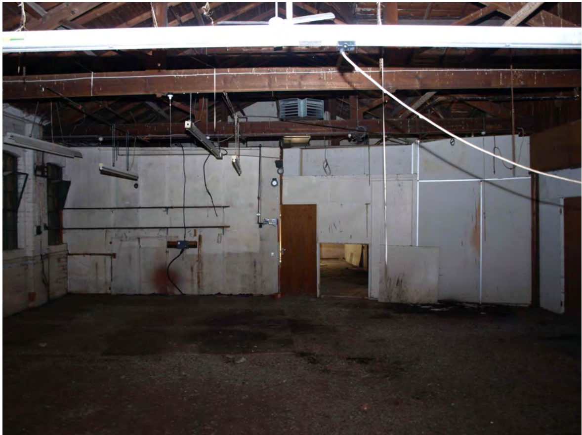
Plate 23: Crude plywood partition dividing up northern wing of original factory
