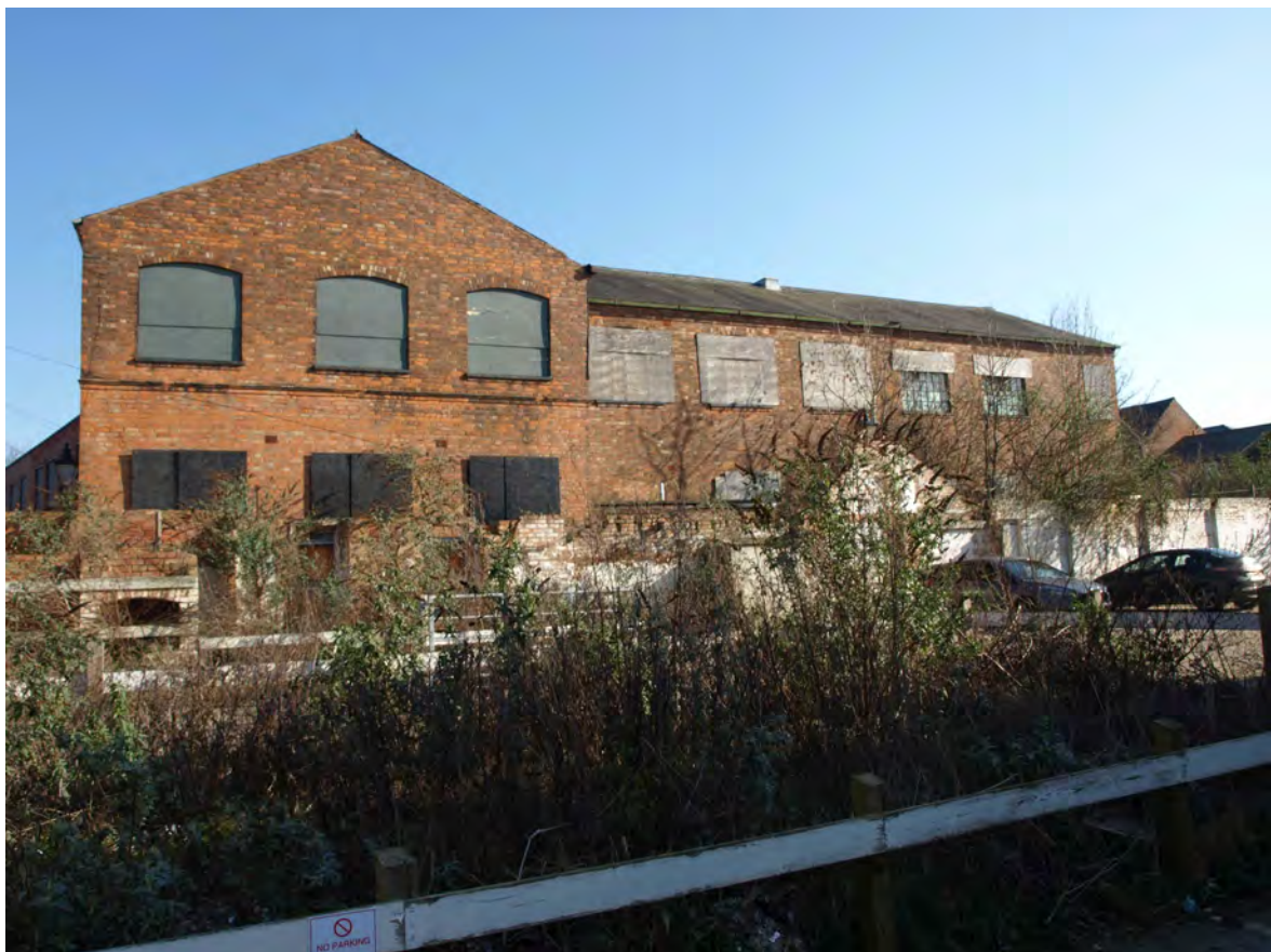
Plate 2: West facing elevation of original T shaped factory
