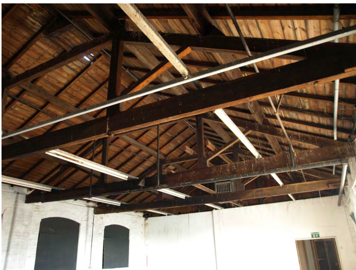
Plate 22: Detail of roof structure
