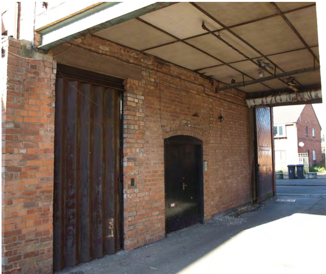
Plate 6: Original east facing gable wall of T shaped factory showing original entrance
