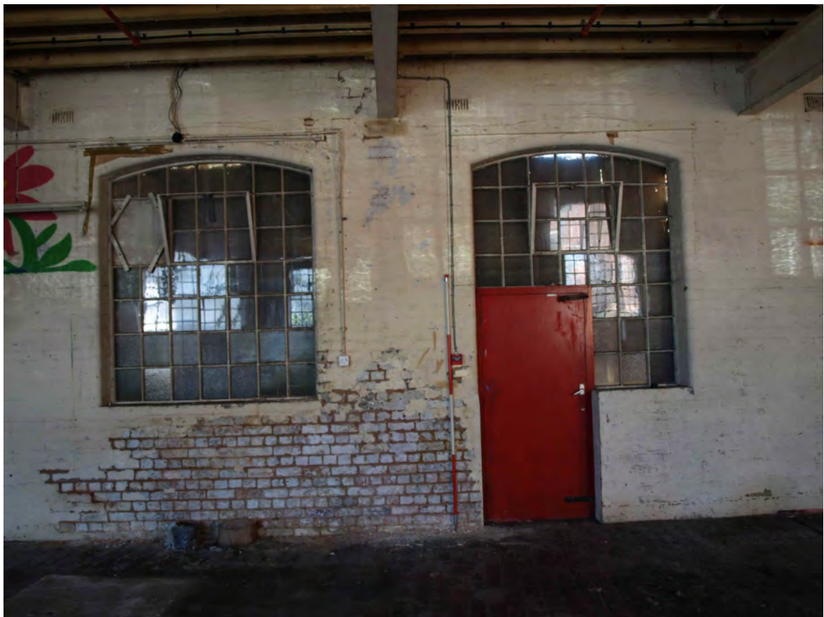
Plate 16: Interior western elevation of south wing showing later door added to allow access to adjacent Jitty
