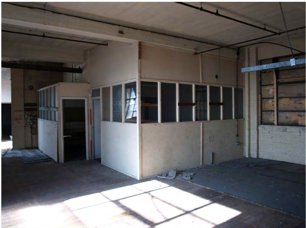
Plate 36: Supervisors' offices in later extension looking north-west
