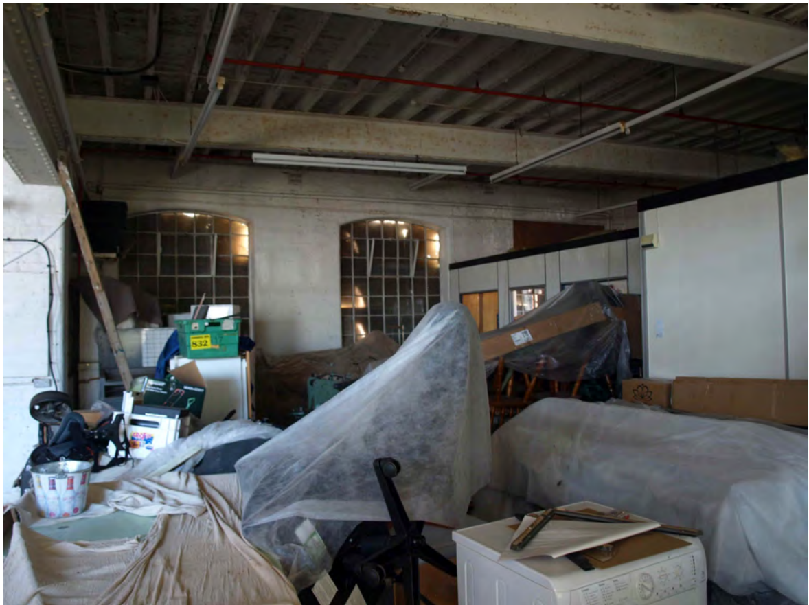
Plate 13: Front northern wing of original factory looking west-north-west
