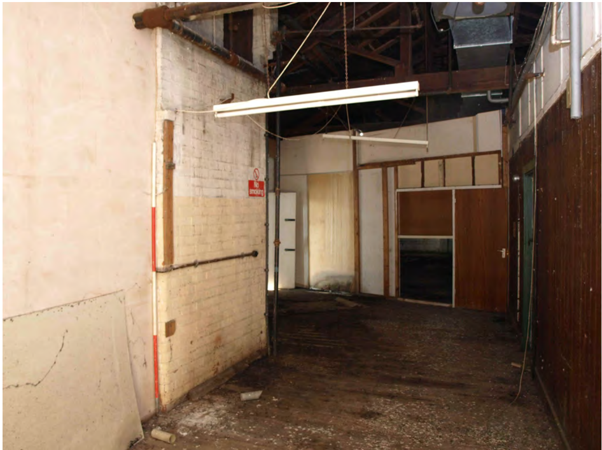
Plate 25: Interface between original factory and new build. The Brick wall on the left shows the point at which the original factory ended and the gable wall opened up on the first floor. Later partitions creating office space can be seen to the right
