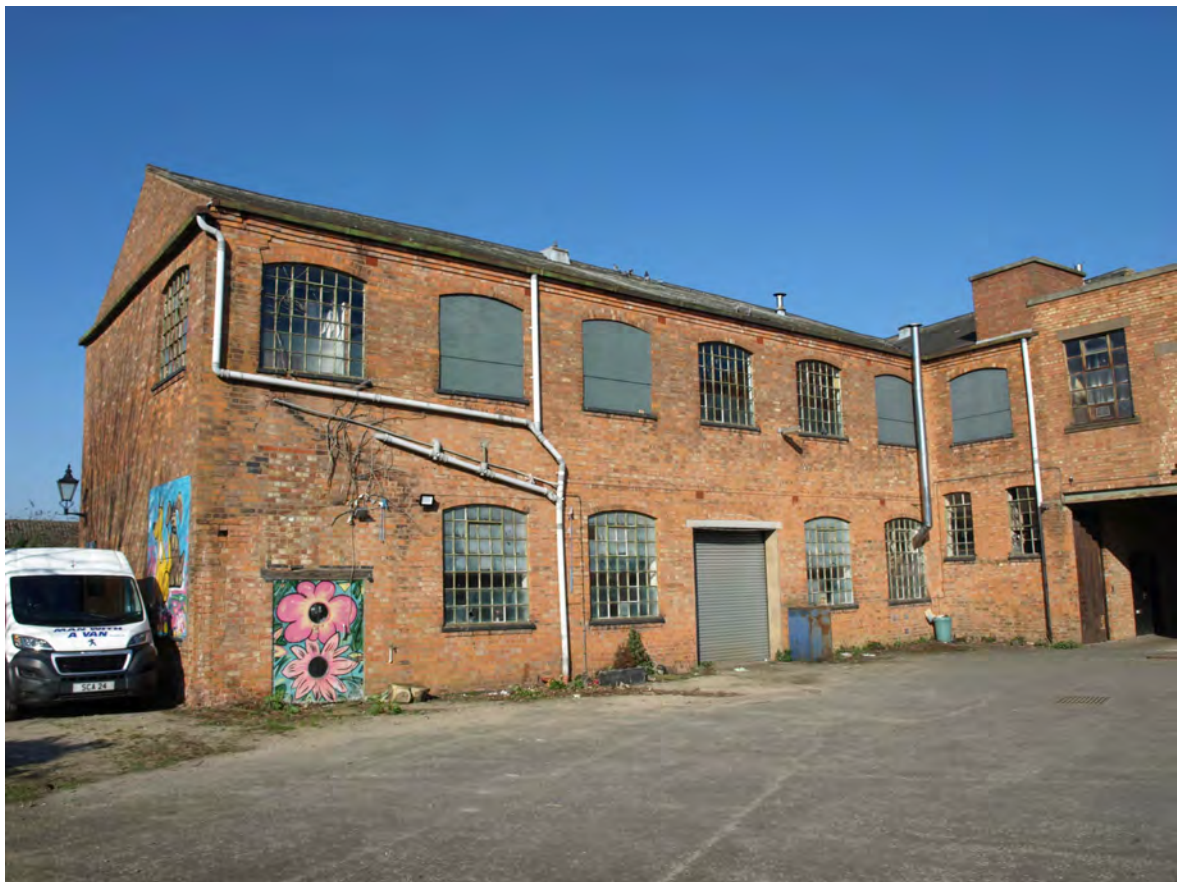
Plate 4: East facing elevation of original T shaped factory
