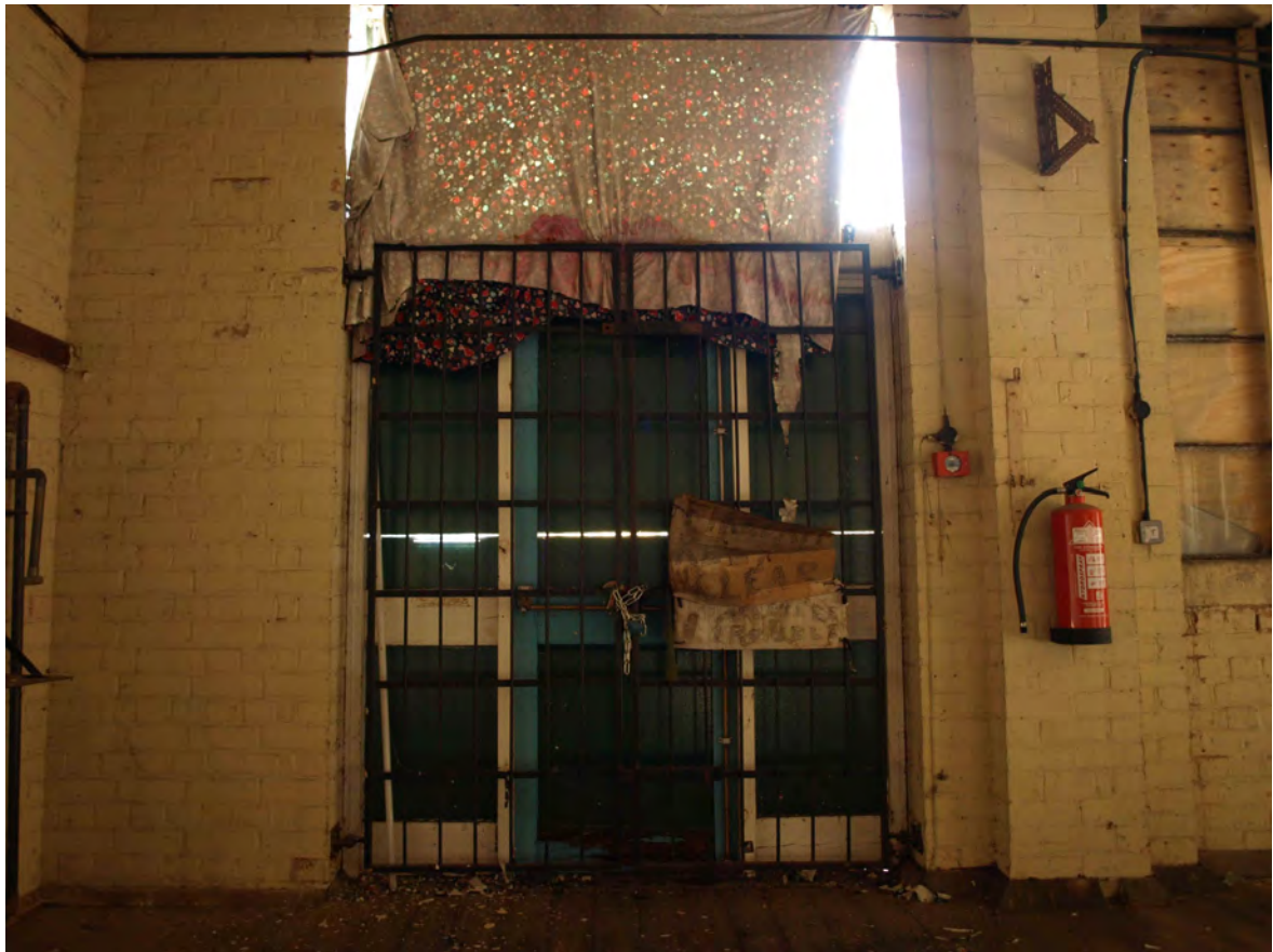
Plate 39: Fire escape located in bay 5
