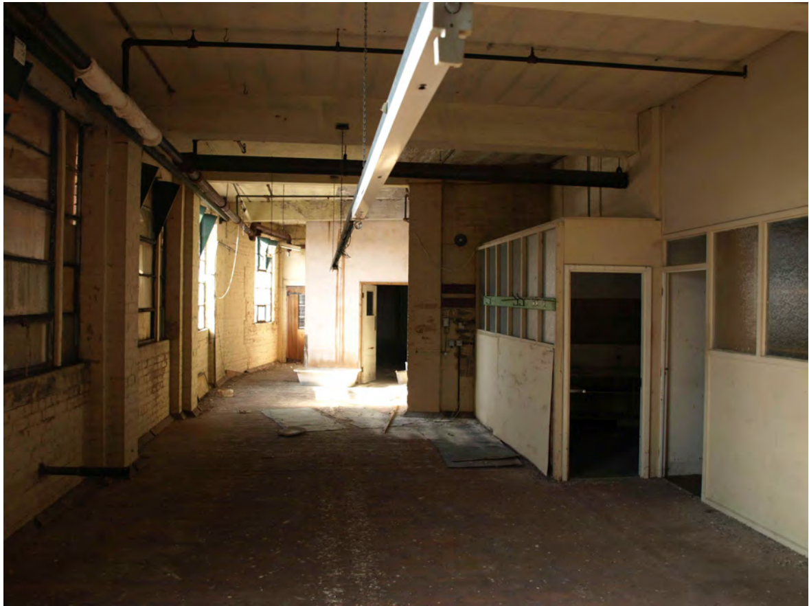
Plate 35: View towards lift and original factory from later extension, probable supervisors' office visible on north side.
