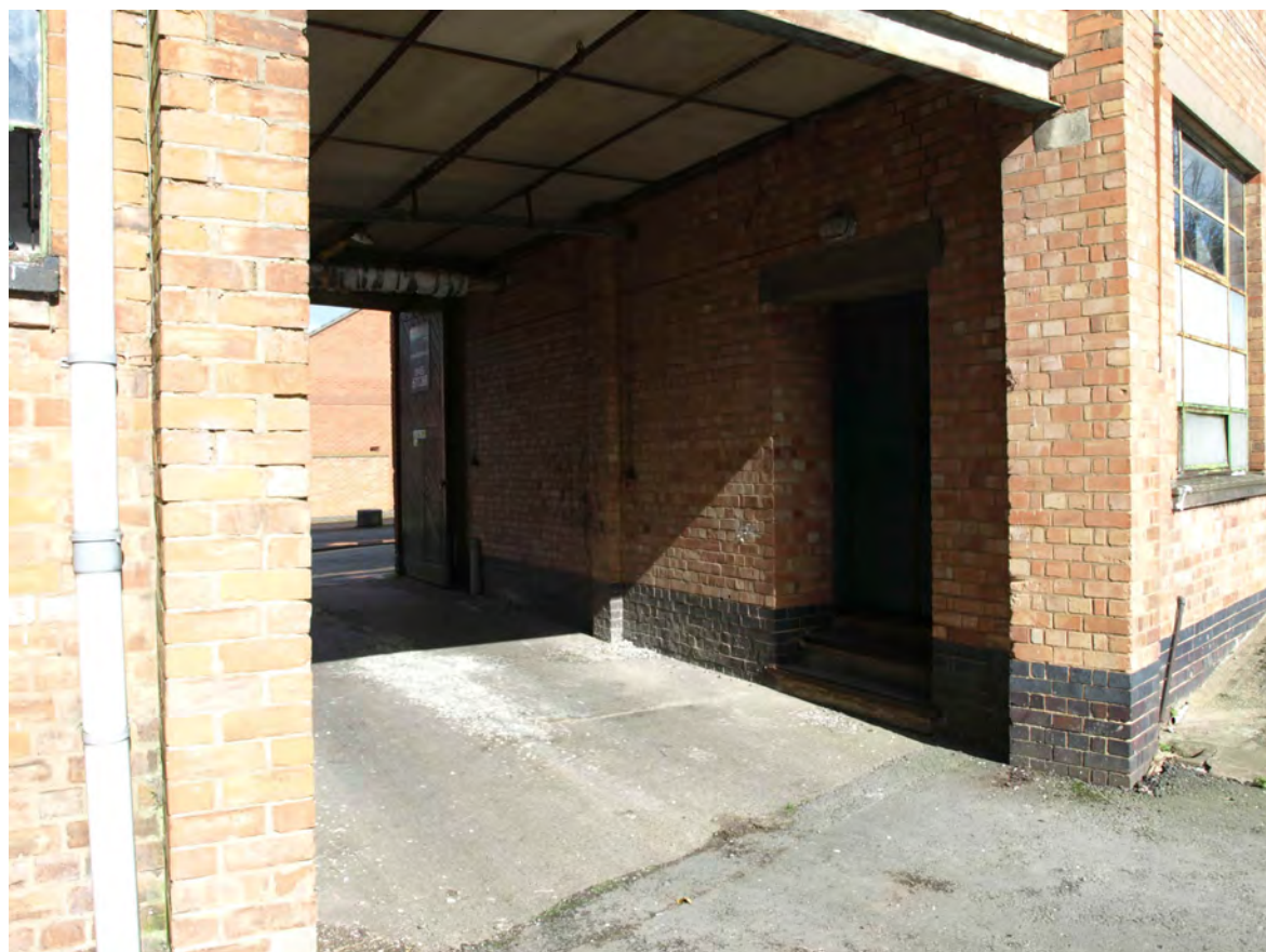
Plate 12: Western side of carriageway showing original door into later extension
