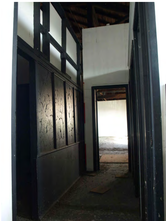
Plate 19: Partitioning showing obscured glass.
