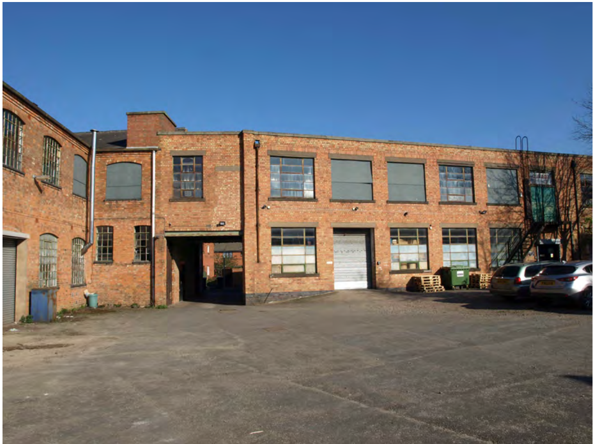
Plate 5: Southern elevation showing interface between original factory and later extension
