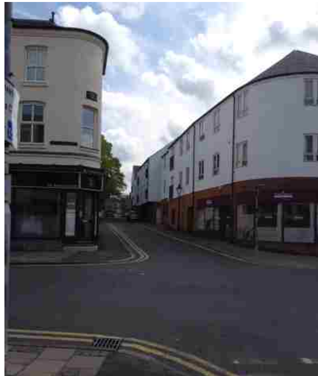
View up Wood Street from junction with New Buildings.
