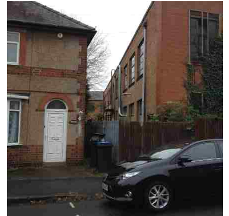
14 note number of large windows in factory overlooking neighbouring house
