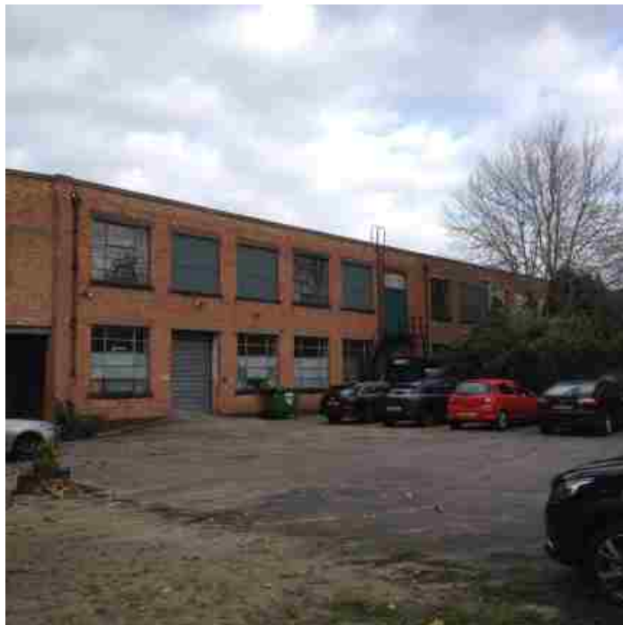
11 rear of factory - note upper floor windows boarded up
