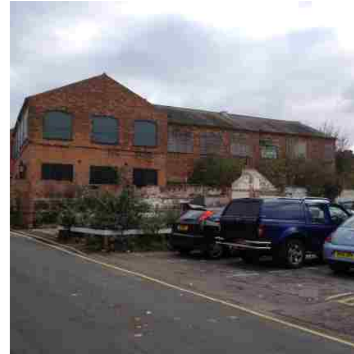
1 empty factory building now in desperate need of repair the cost of which has made it unviable
