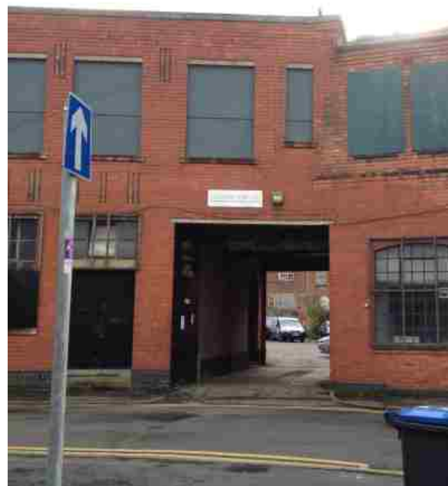
Existing access into site very tight with inadequate visibility for vehicles leaving site - particularly hazardous for pedestrians crossing.
