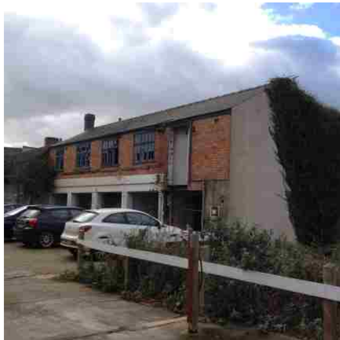
3 the derelict building referred to in photo 2 has now been sold and is in the process of being renovated
