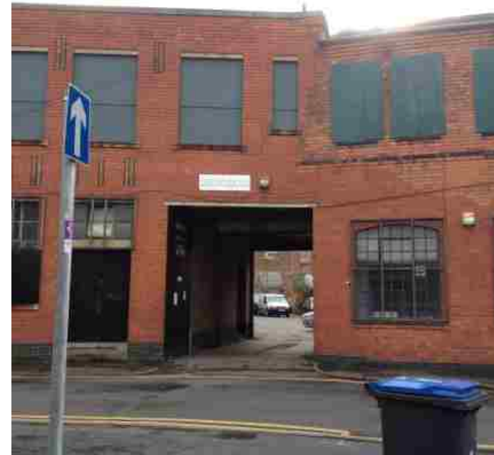
9 junction between the two factory elements showing the only access to the rear car park and service area - the width and poor pedestrian visibility makes it unsuitable for service vehicles
