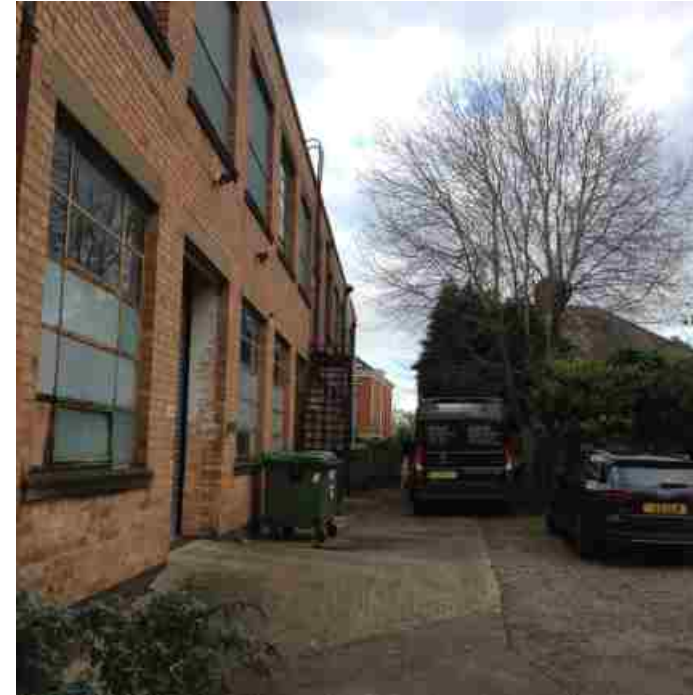
13 view through gap between factory and house - dense hedge screening on boundary helps privacy
