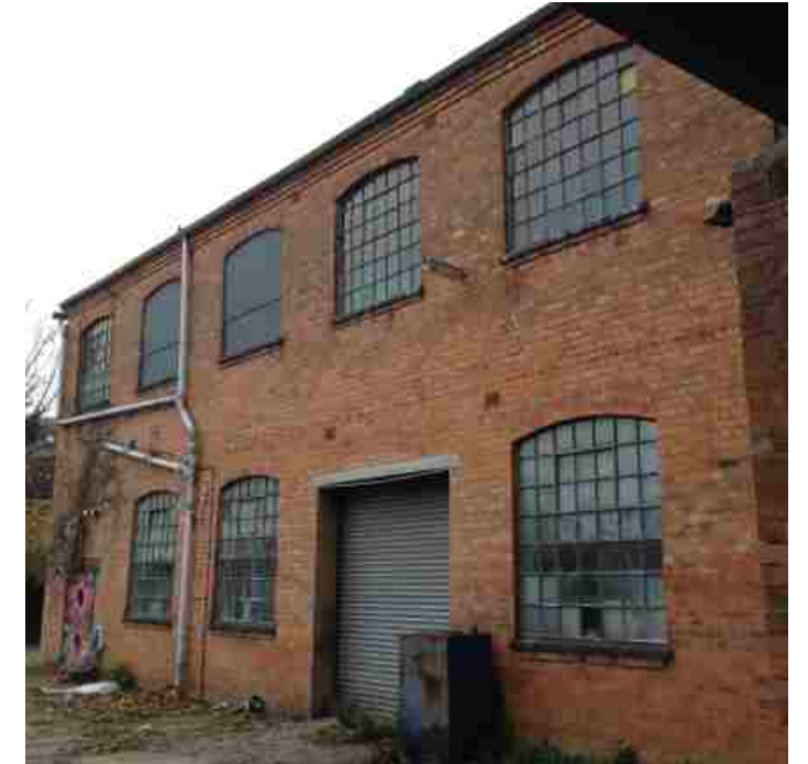
10 rear of original building with original single glazed metal windows - roller shutter door a later addition
