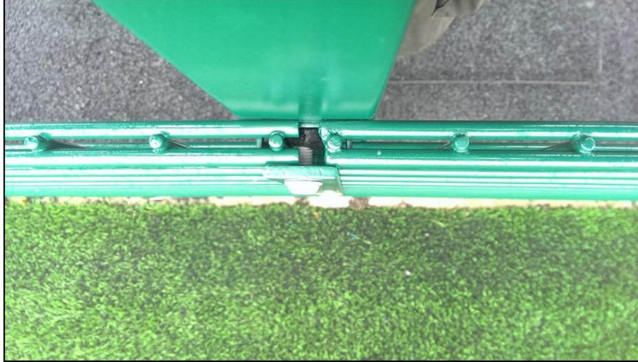
Figure 8: Image Showing Neoprene Isolators
