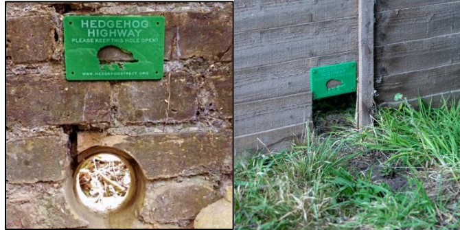
Figure 16: Examples of hedgehog highways in a brick wall (left) and wooden fence (right)
