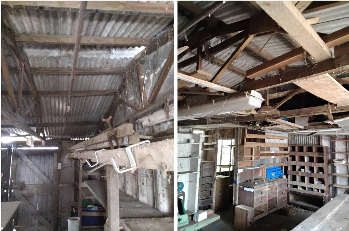
Photos 7 + 8. Internal structure of the garage building.
