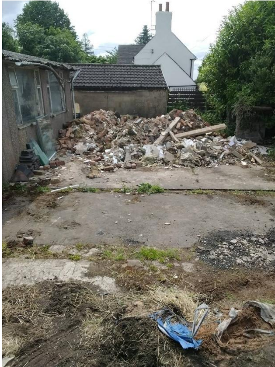
Photo 5. Asphalt and concrete slab driveway.
