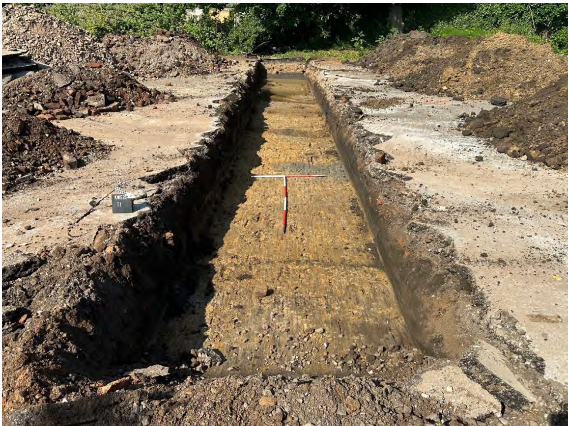
Plate 4: Trench 2 looking south-west
