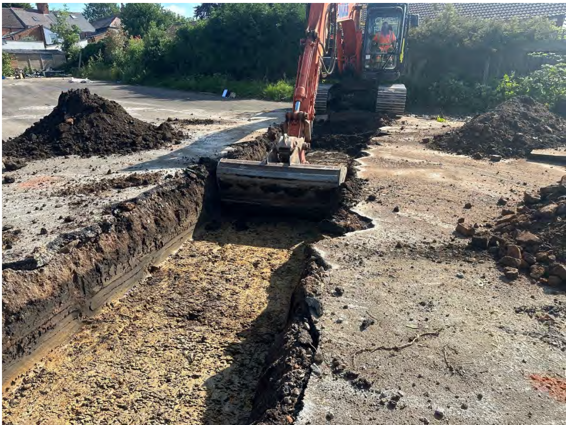
Plate 2: General view of excavation in progress
