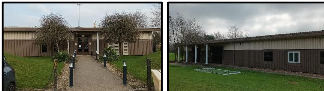
Figure 6: Southern and Western Elevations of B1.
