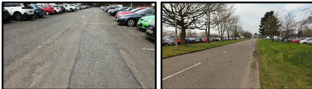
Figure 4: Example of Developed Land; Sealed Surface.
