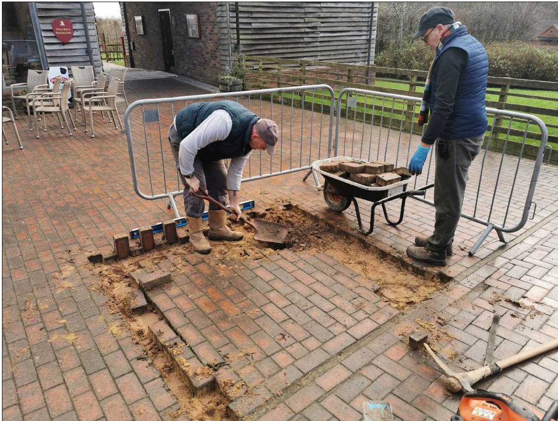
Figure 5: Exposing sand blinding below brick paving, looking south-east
