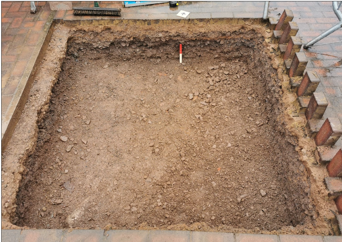
Figure 7: Excavated foundation pit, showing aggregate continuing below base, looking north (0.2m scale)
