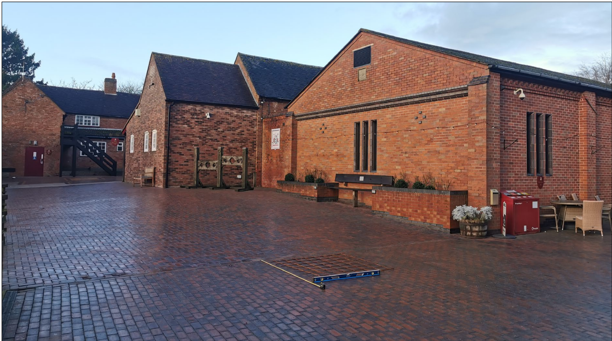
Figure 3: Area of proposals prior to groundworks commencing, looking north-west
