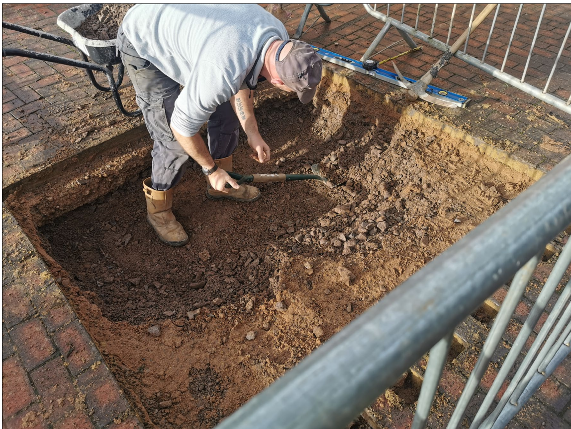
Figure 6: Excavating aggregate base, looking north-west
