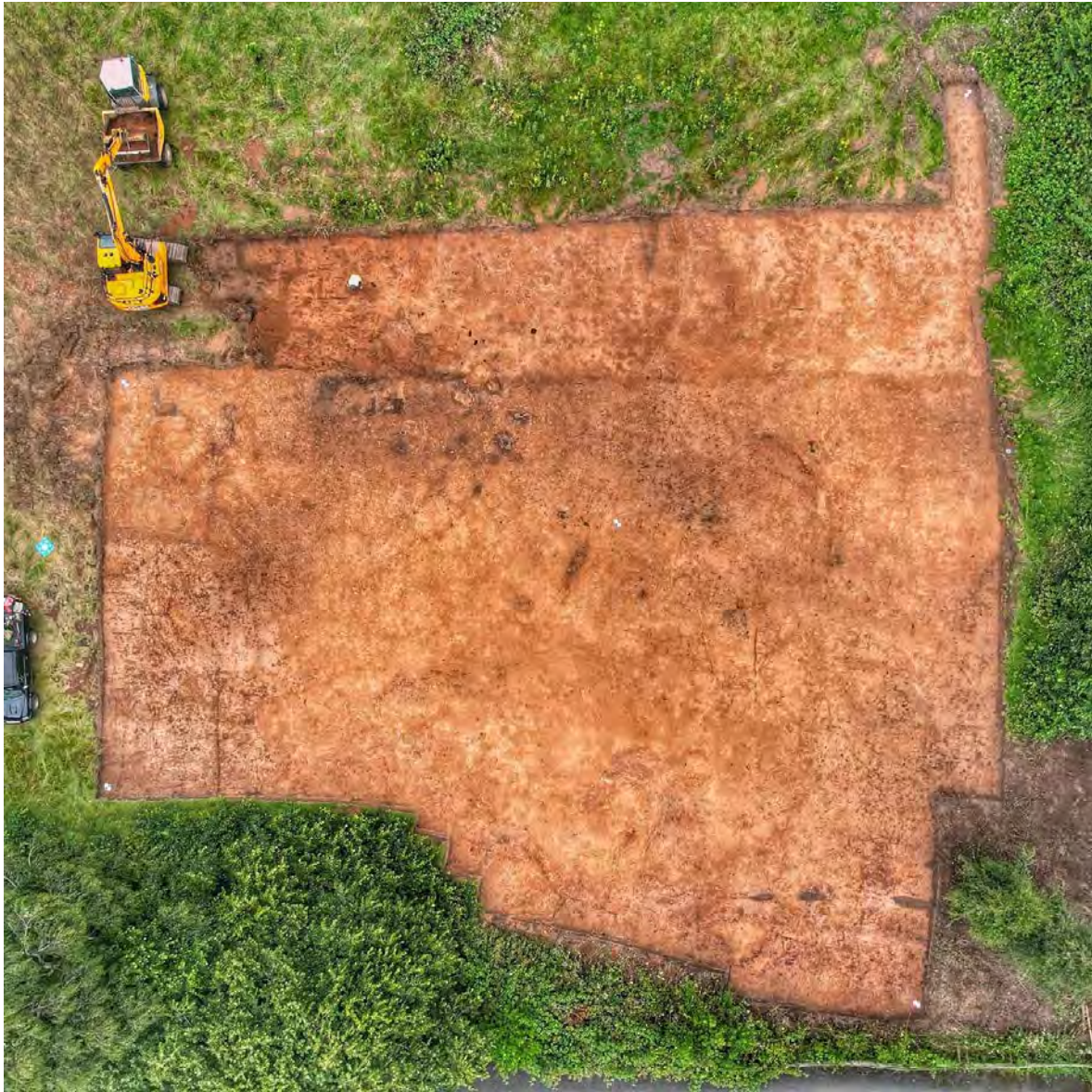
Plate. 1 Aerial View of Strip in Progress
