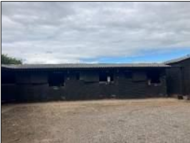
Figure 31: Small timber and corrugated roofed stable - well maintained and in-use.
